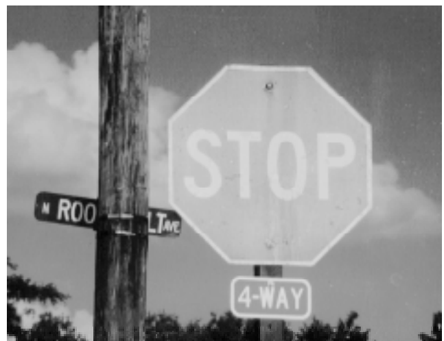
Stop sign in poor condition Note: Street sign is improperly placed.
