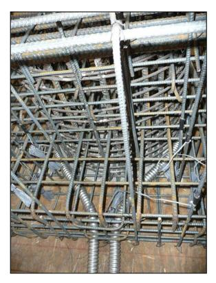
Figure 5.10: Placement of Ducts in the Bent Cap around the Column
