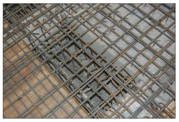
Figure 5.12: Partial Diaphragm Pour between Girders
