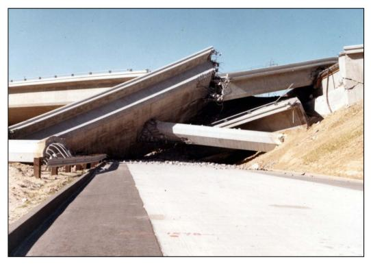
Figure 1.1: Example of 1971 San Fernando Earthquake Damage (Courtesy of UCSD)
