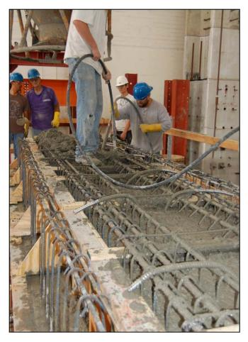
Figure 5.8: Casting of the Bent Cap
