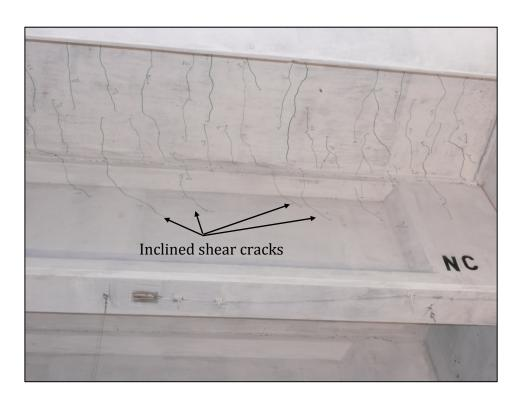
Figure 6.30: Inclined Shear Cracking Observed on the Center Girder on the Improved Connection Side at
