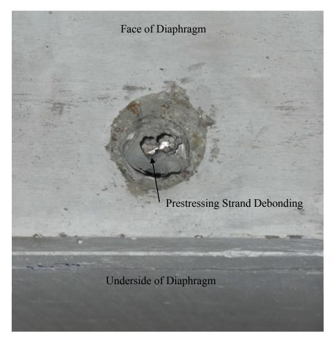
Figure 5.13: Untensiond Strand Debonding
