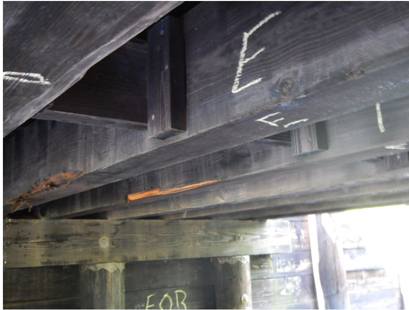
Figure 6-5 Stringer damaged by debris strike
