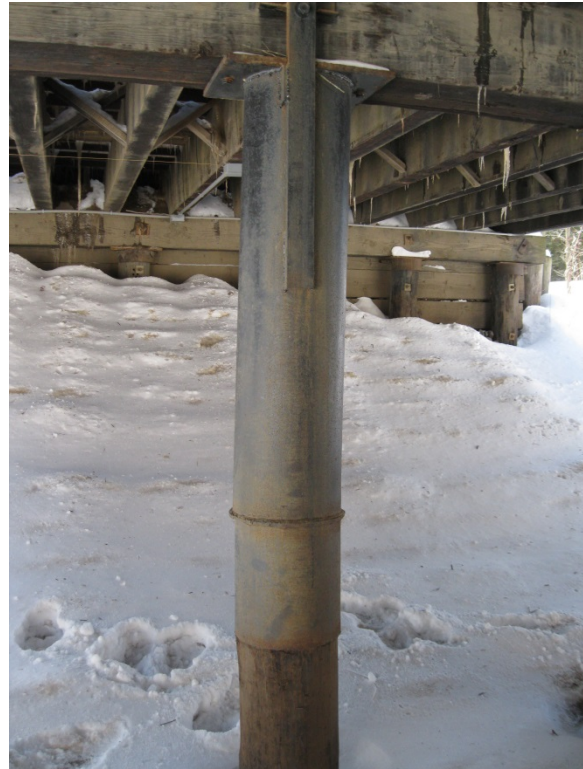
b) Steel replacement of timber pile
