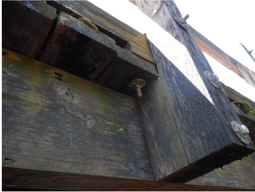
Figure 6-6 Staining and vegetation growth
