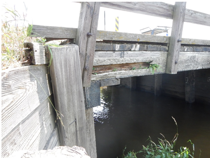
Figure 6-7 Moderate decay along face of exterior girder
