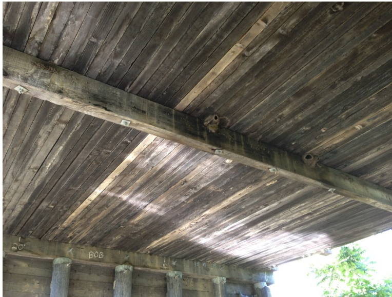
Figure 8-1 Repair of laminated decks
