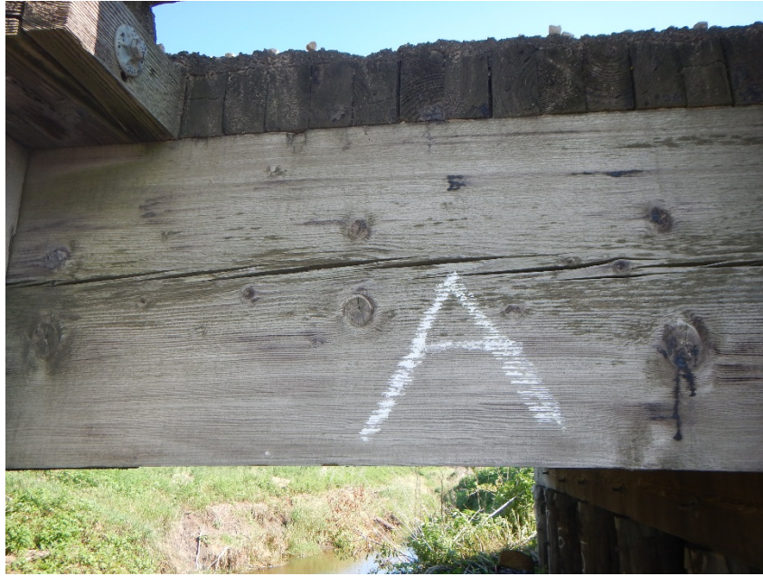
Figure 6-8 Checking at mid-depth of exterior girder
