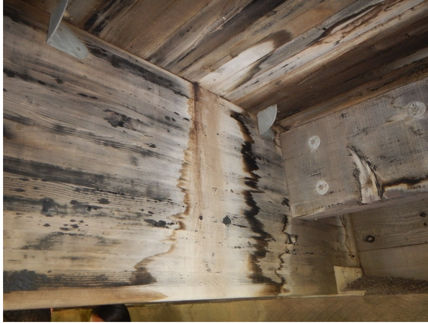
Figure 6-3 Localized deck drainage through asphaltic wearing surface
