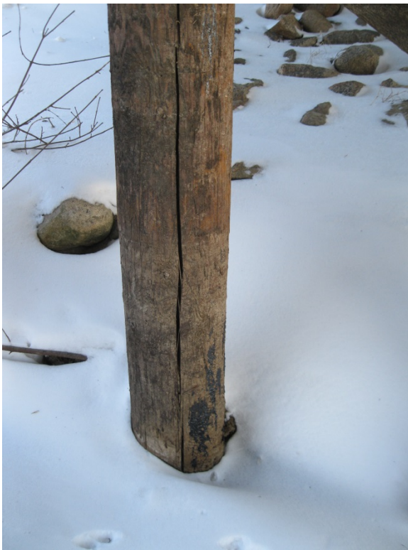
a) Large check in pile at waterline
