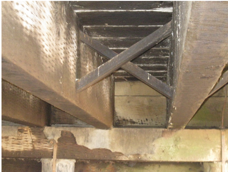
Figure 8-9 Strengthening of individual timber stringers
