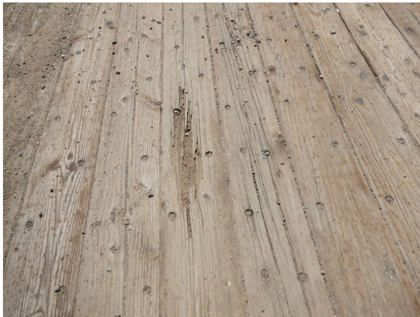
Figure 6-1 Timber deck without wearing surface in apparently good condition overall
