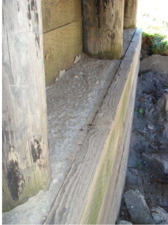
Figure 3-19 Timber planking and concrete encapsulation
