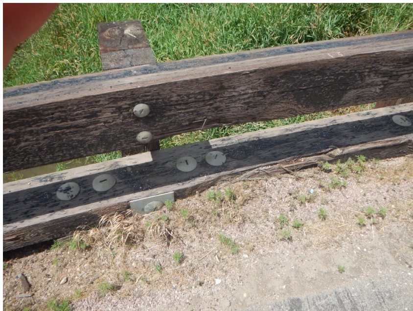
Figure 6-4 Deck debris accumulation at deck edge
