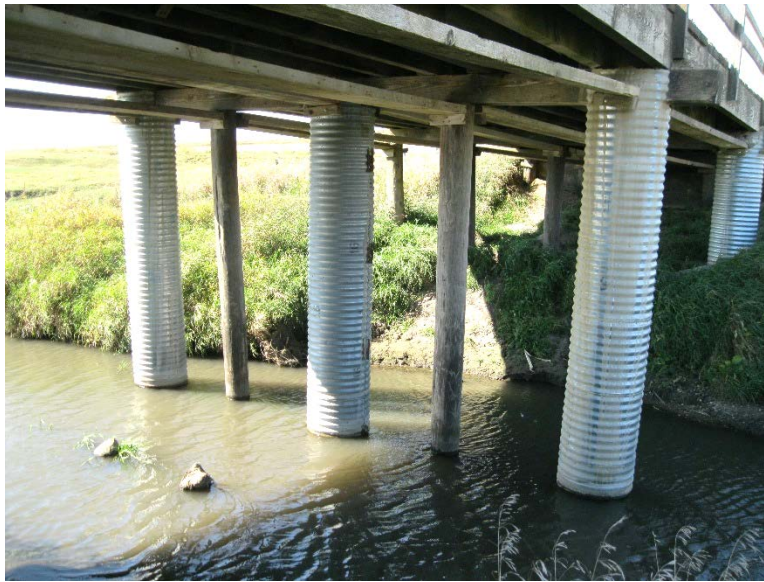
Figure 8-16 Addition of pile jackets
