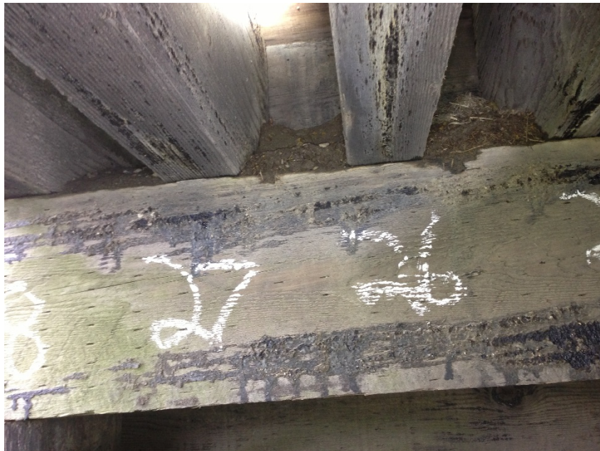
Figure 6-9 Debris accumulation between stringer ends and pile cap
