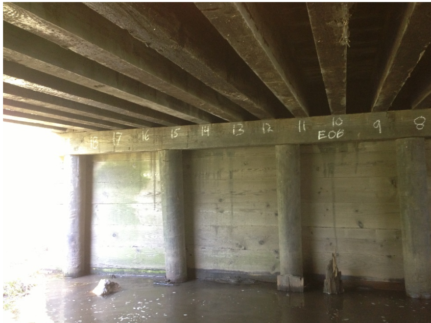
Figure 2-2 Typical stringer/multi-beam or girder bridge
