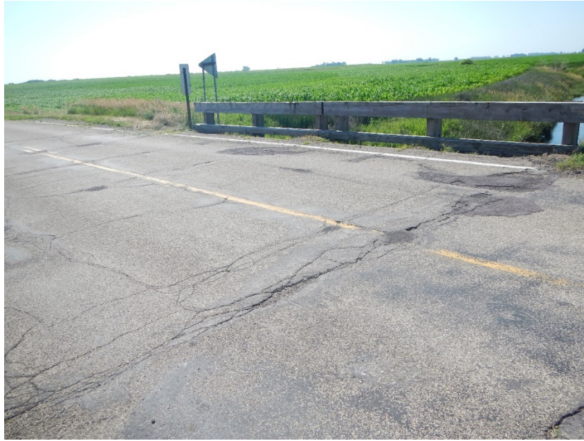
Figure 6-2 Cracking of asphalt wearing surface
