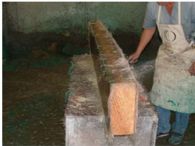
Figure 3-28 Sprayed fiber-reinforced polymer
