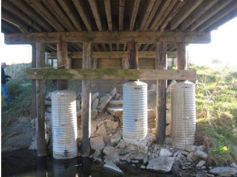
Figure 3-10 Concrete jacketing using corrugated metal pipe
