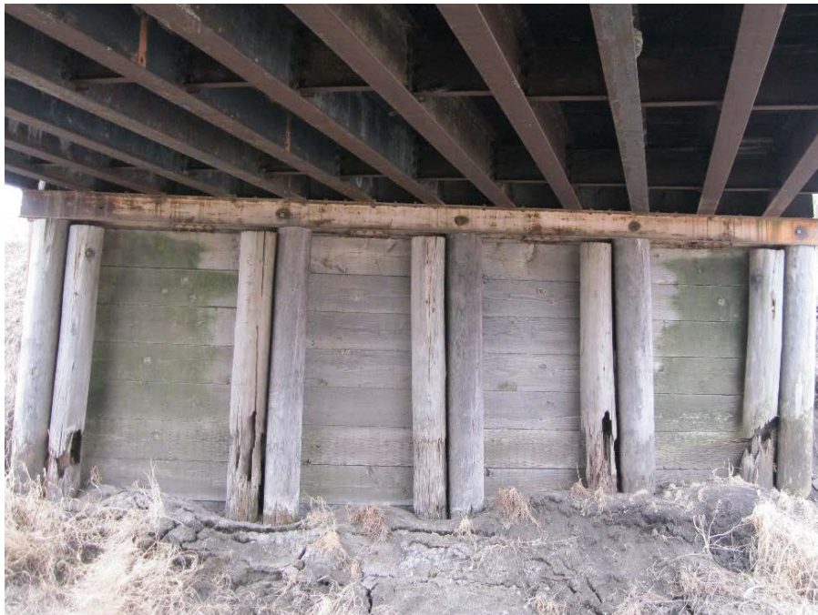
Figure 6-12 Severely decayed timber piles at abutment
