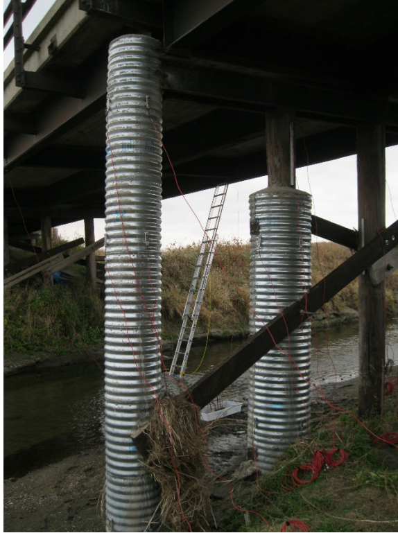
Figure 7-1 Concrete jacketing in CMP
