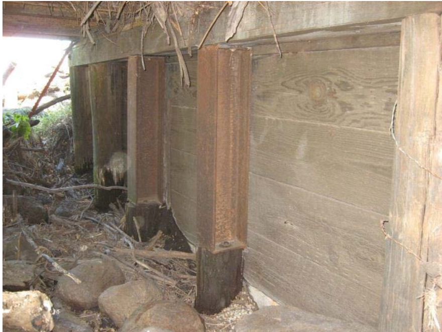
Figure 3-2 Posted piles using steel W shapes
