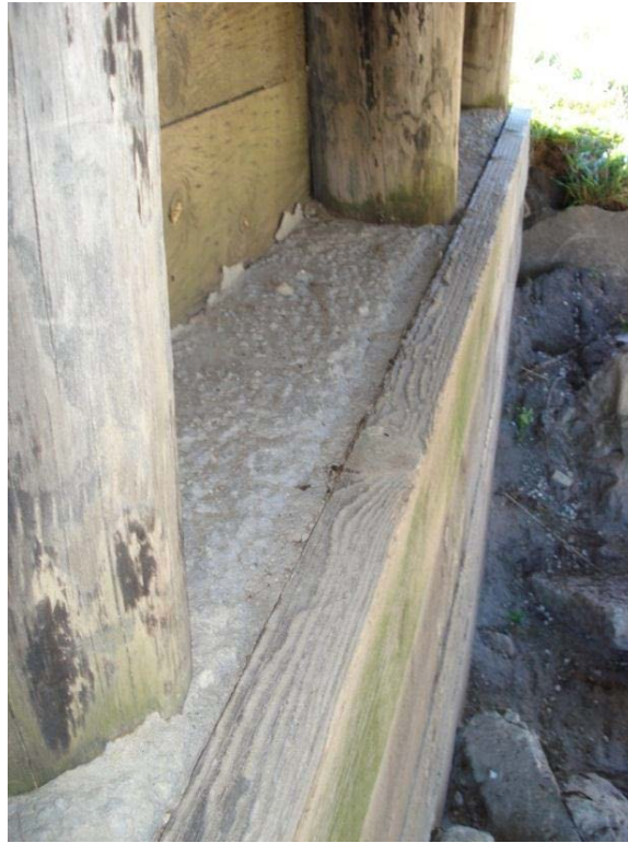
Figure 7-2 Pile encapsulation with timber planks and concrete
