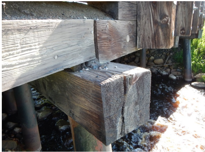
Figure 6-13 Advanced checking in pile cap
