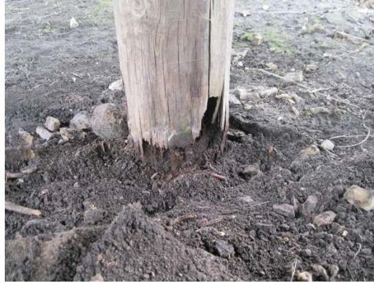
Figure 6-11 Advanced decay at the ground surface
