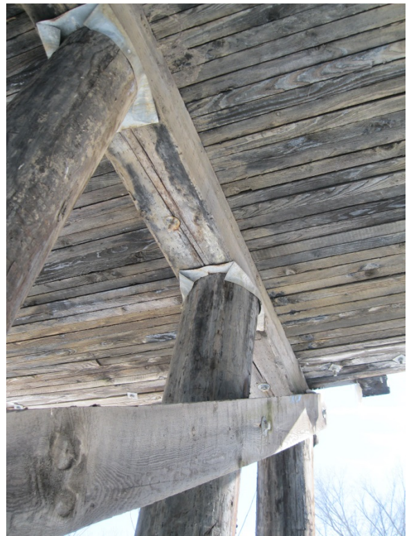
b) Large checks in pile cap
