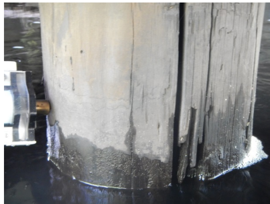
Figure 6-10 Pile splitting at the waterline
