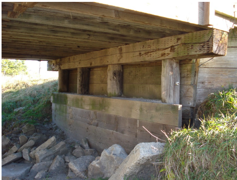
Figure 8-18 Pile encapsulation at abutment
