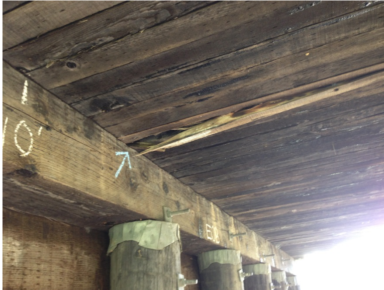
Figure 7-4 Localized deterioration and damage in laminated timber deck
