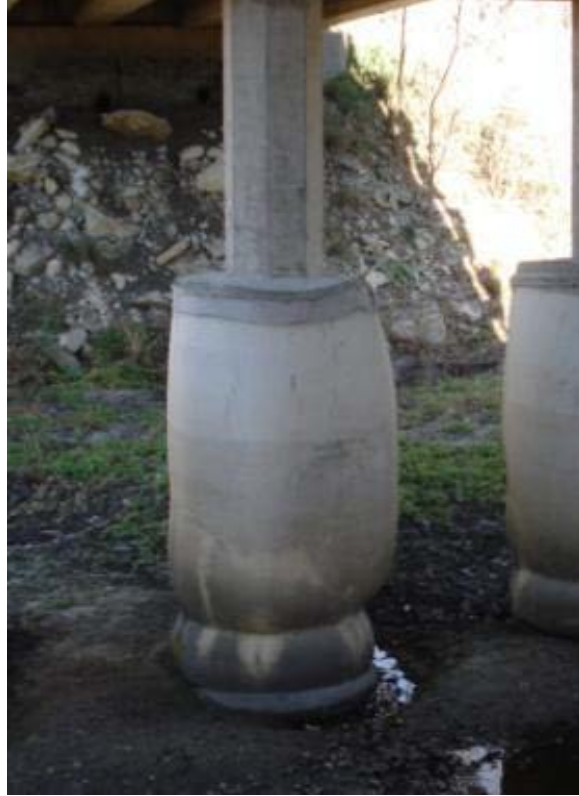
Figure 3-11 Concrete jacketing with nylon sock
