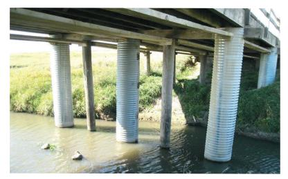
Concrete pile jackets—concrete-filled steel shells installed to strengthen timber piles weakened by minor to moderate deterioration—are one of the rehabilitation procedures detailed in the timber bridge repair manual.
