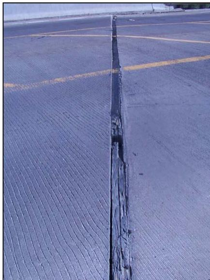
**(a) Deteriorated joint filler**
