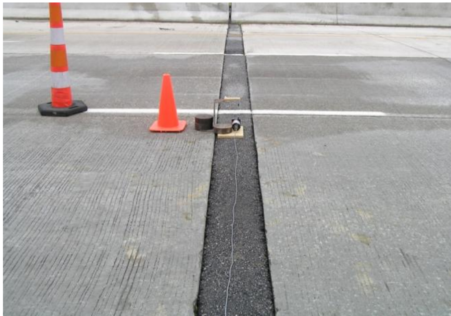
Figure 5.45. 12 in. pressure relief joint condition
