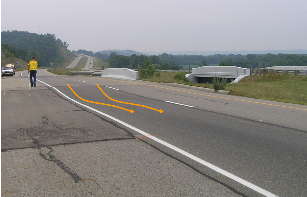
Figure 5.17 Dip in pavement when exiting the bridge
