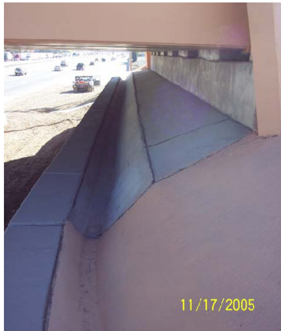
Figure 4.37. Drainage gutter used in New Mexico for moving water away from the bridge embankment (Lenke, 2006)
