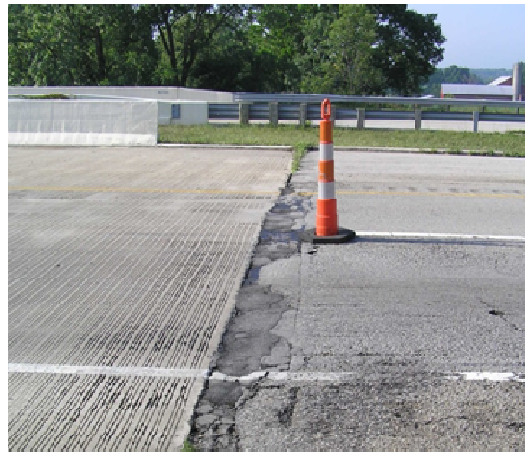
b. Approach-to-pavement joint
