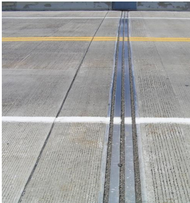
b. Approach to bridge joint
