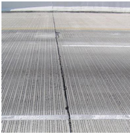
a. Approach-to-bridge joint
