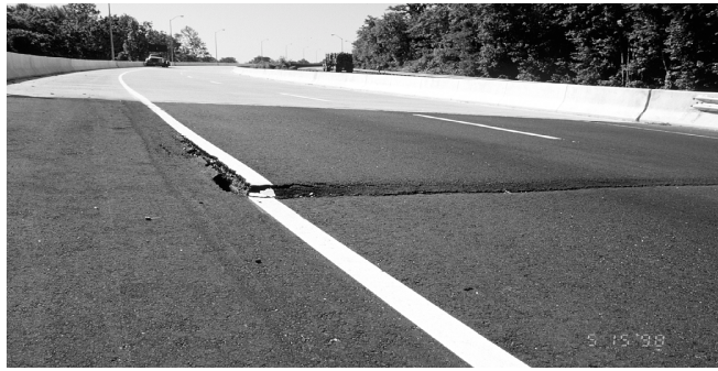
Figure 4.60. Approach slab distress attributable to foundation soil settlement (Route 10 westbound lane over the Appomattox River) (Hoppe, 1999)
