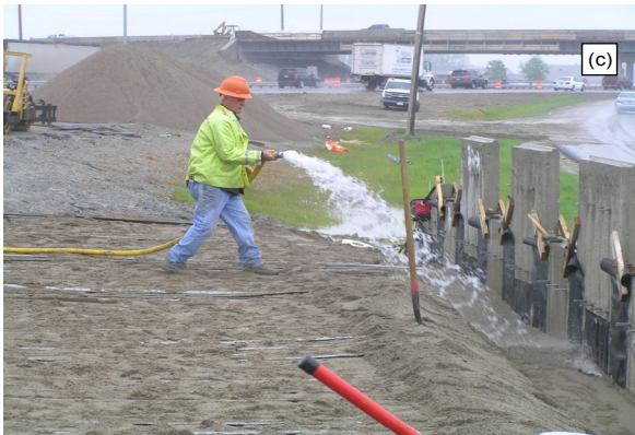
c. watering of backfill prior to compaction
