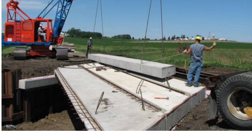
Figure 4.6. Setting panel on superstructure
