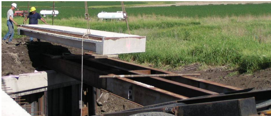
Figure 4.4. Temporary beams for setting panels
