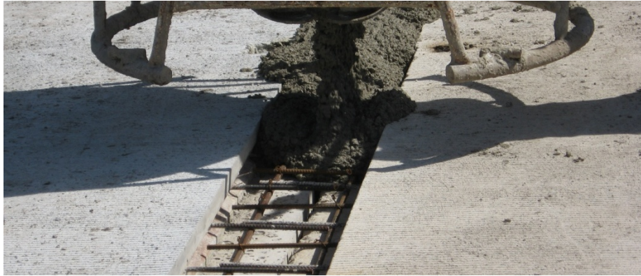
Figure 4.15. Concrete in closure area
