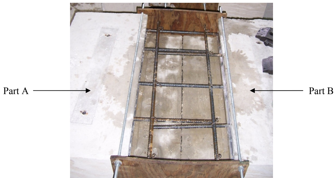
Figure 2.16. Position of reinforcing bar before closure
