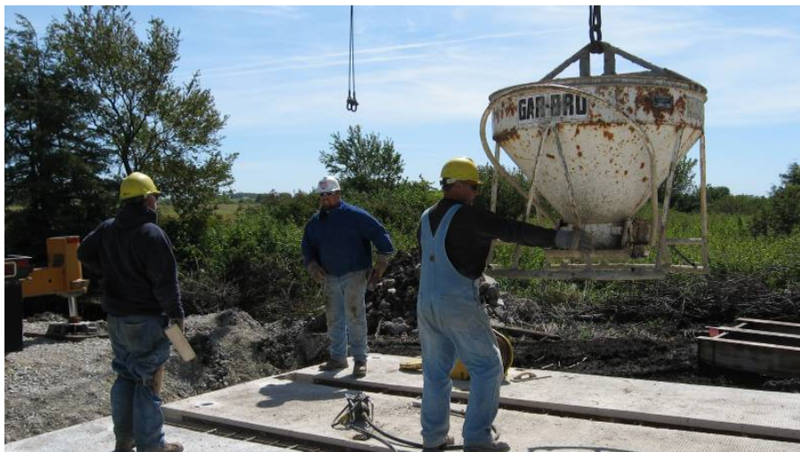
Figure 4.14. Using concrete bucket for placement
