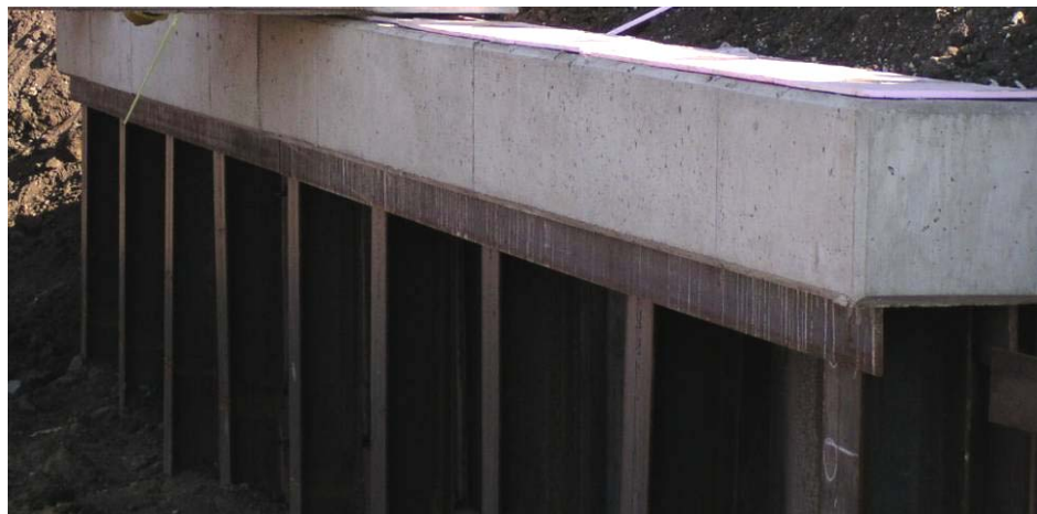
Figure 4.3. Abutment cap on H-piles
