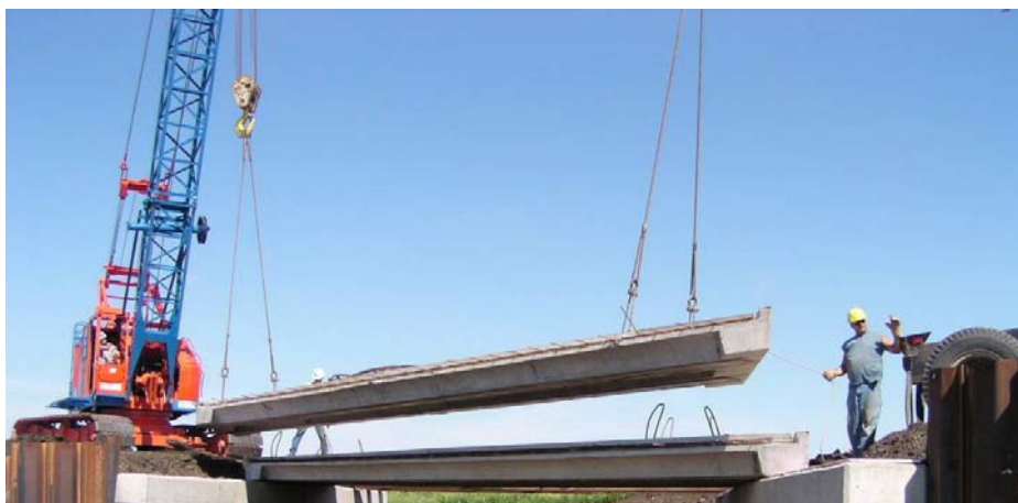
Figure 4.5. Using two cranes to position a deck panel
