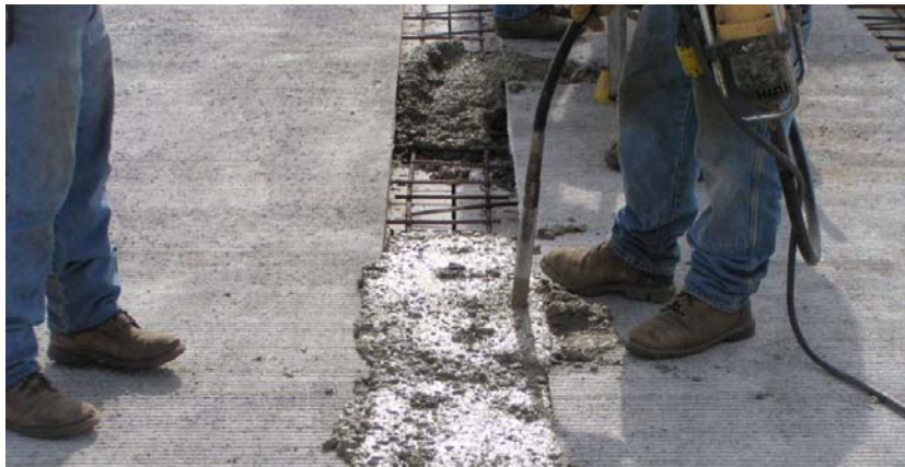
Figure 4.8. Closure concrete placement
