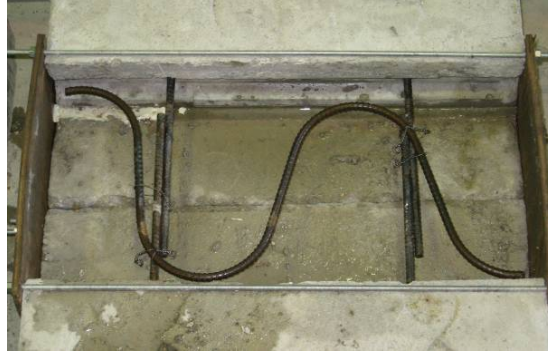
Figure 2.25. Formwork for closure in Type 3 Connection
