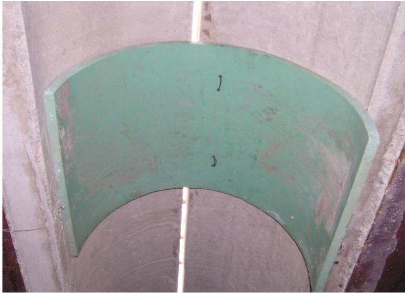
Figure 4.7. PVC form used in the location of a gap between the concrete panels
