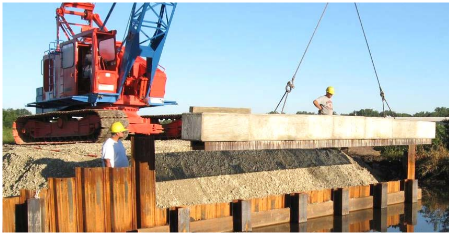
Figure 4.13. Placement of the precast abutment cap for the MRB
