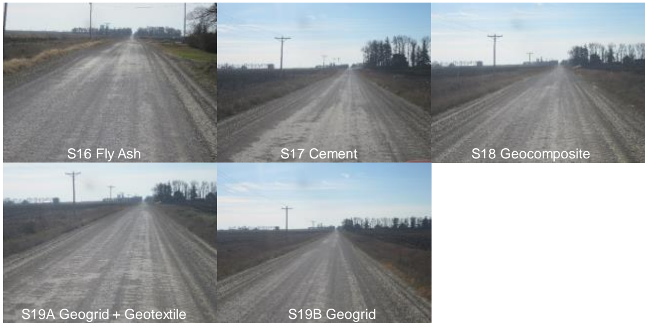
Figure 17. Survey photos of Sections 16 through 19B taken on November 21, 2016
