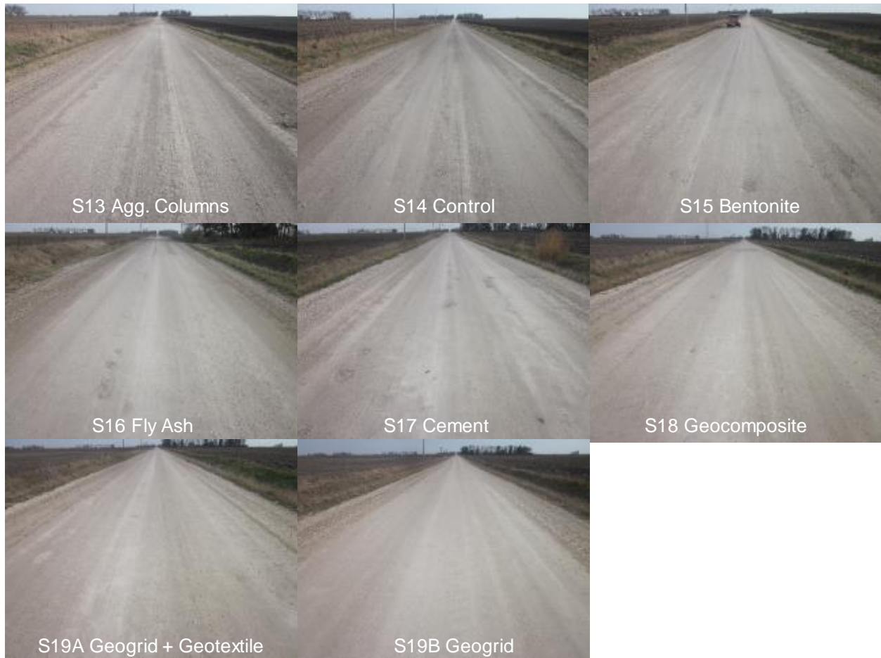
Figure 23. Survey photos of Sections 13 through 19B taken on April 8, 2017
