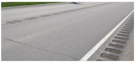
Reflective cracks in non-interlayer overlay on US 169 in April 2014
