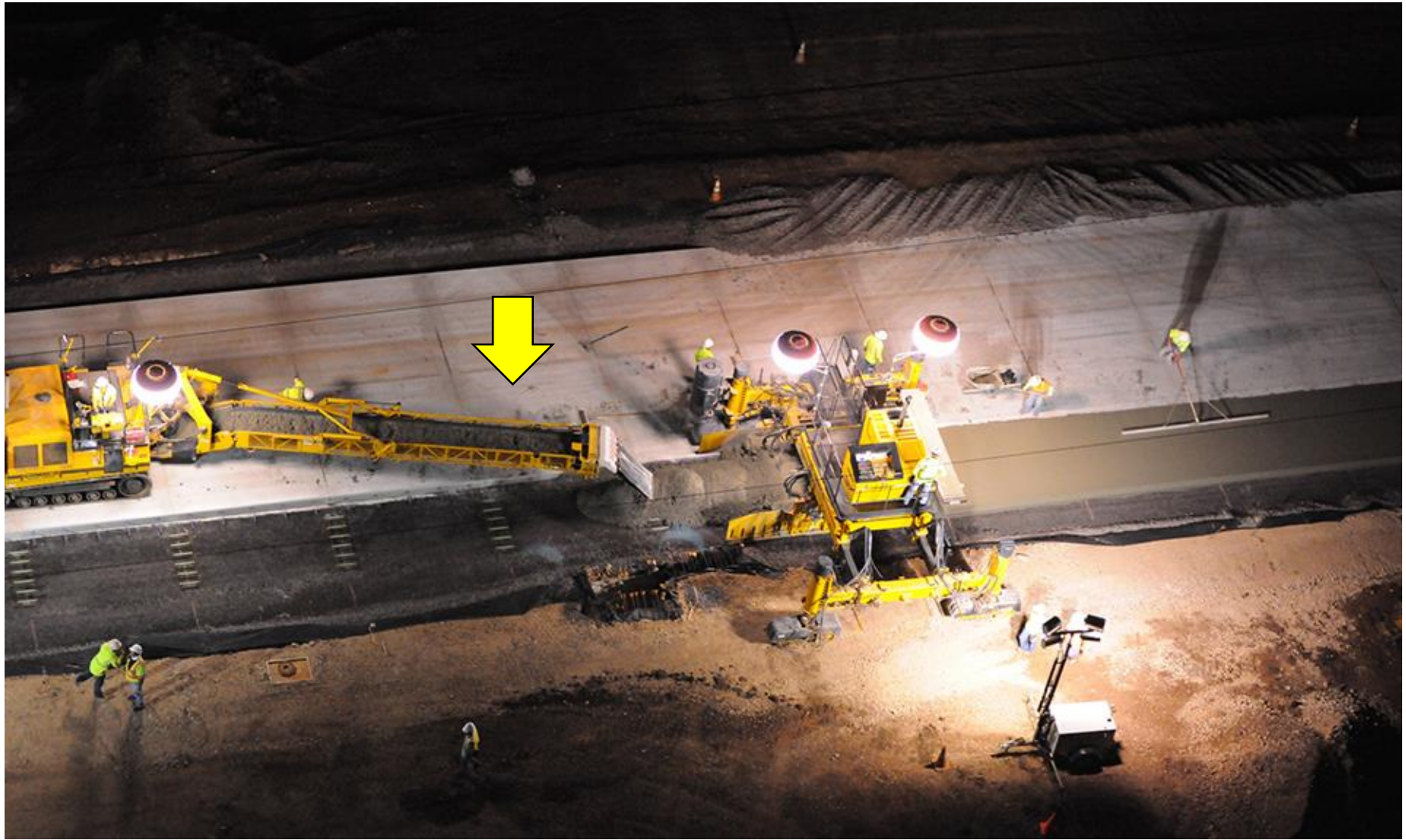
Placer spreads concrete ahead of paver (nighttime construction).
