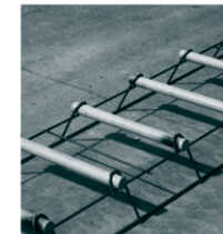
Figure 1. Typical dowel basket assembly
