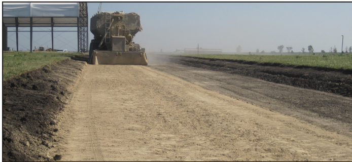
Figure 2. Spreading Ames FA on the 12th St. North section
