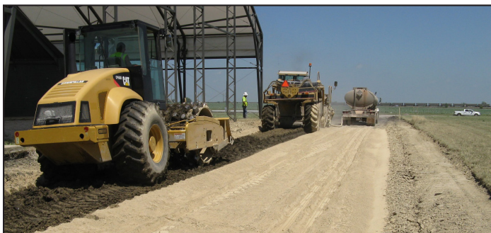
Figure 4. Compaction of subgrade mixed with Port Neal FA on 12th St. North using a padfoot roller
