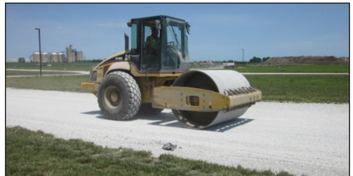
Figure 5. Compaction of a crushed limestone subbase layer using a vibratory smooth drum roller
