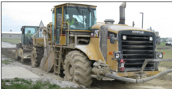
Figure 3. Mixing and moisture-conditioning Port Neal FA with subgrade on the 11th St. South section using a soil reclaimer
