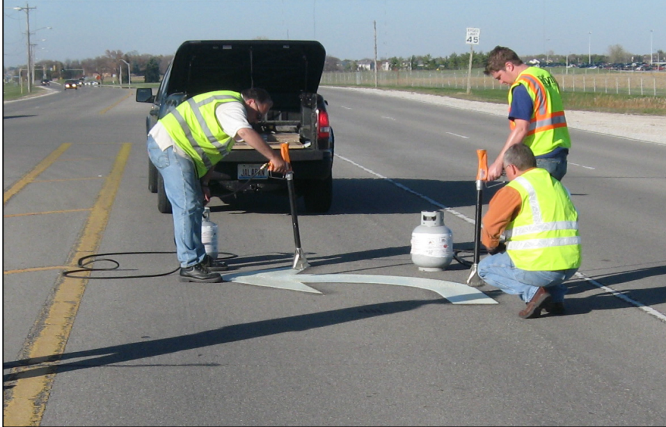
October 2008 – Rural Left Turn Arrow Installation ( R_L=404 ), on asphalt.
