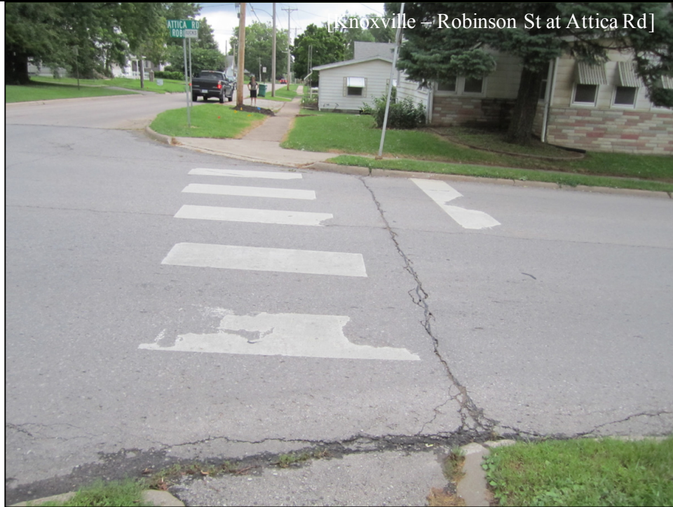
July 2010 – Thermoplastic after 12 months (Stop bar and Crosswalk placed on the south leg of the intersection. Presence=Pass.
