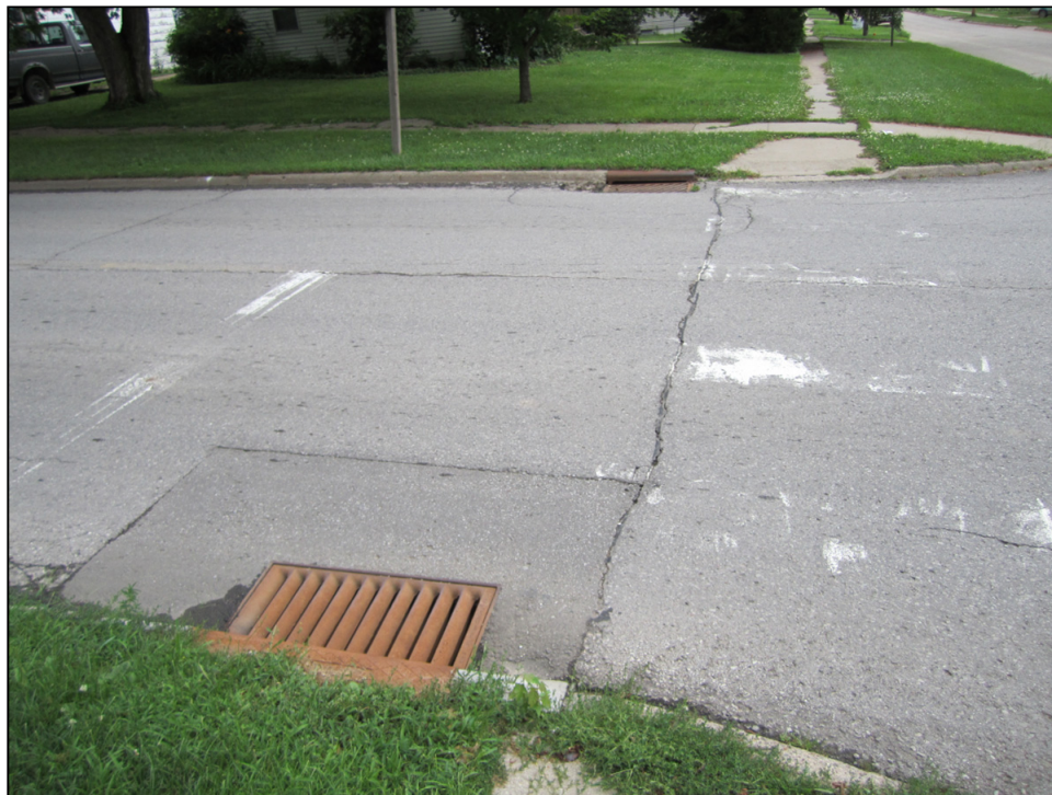
July 2010 – Waterborne Paint after 12 months (Stop bar and Crosswalk placed on the north leg of the same intersection as above. Presence=Fail.
