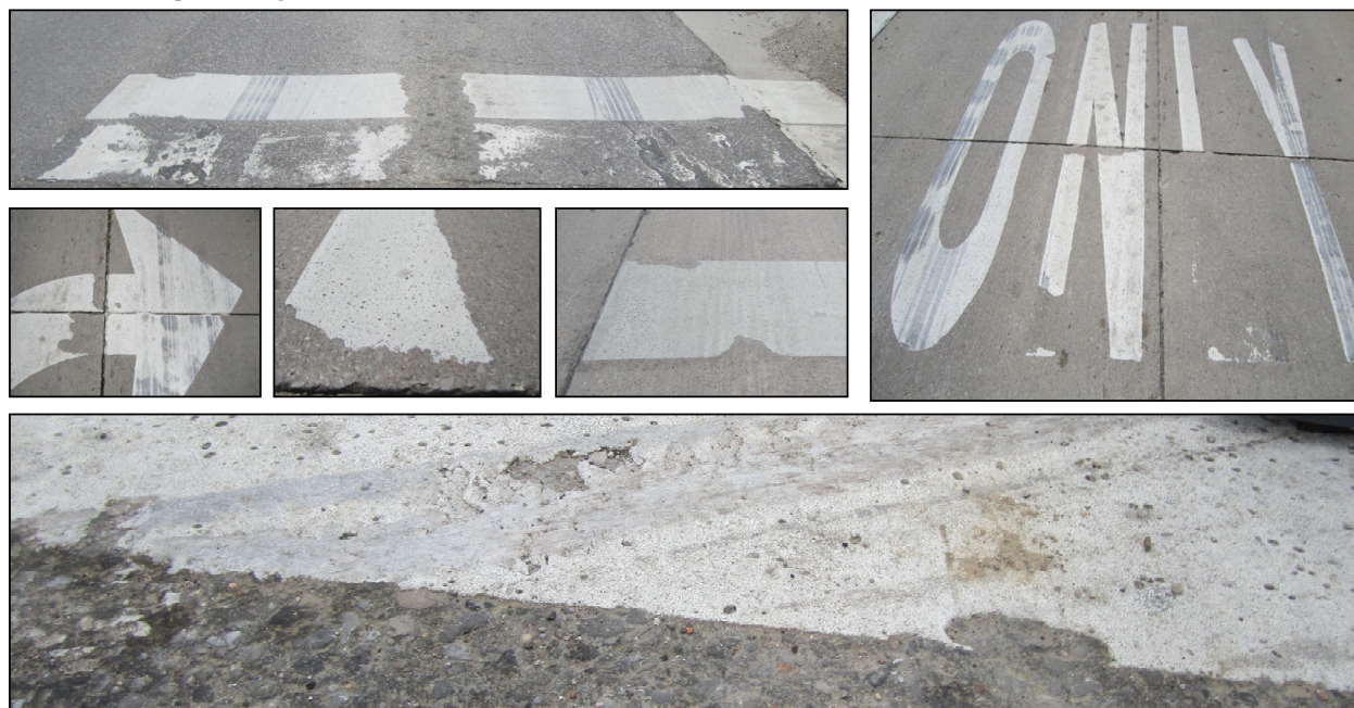
Figure 35. Transverse marking installation and performance
