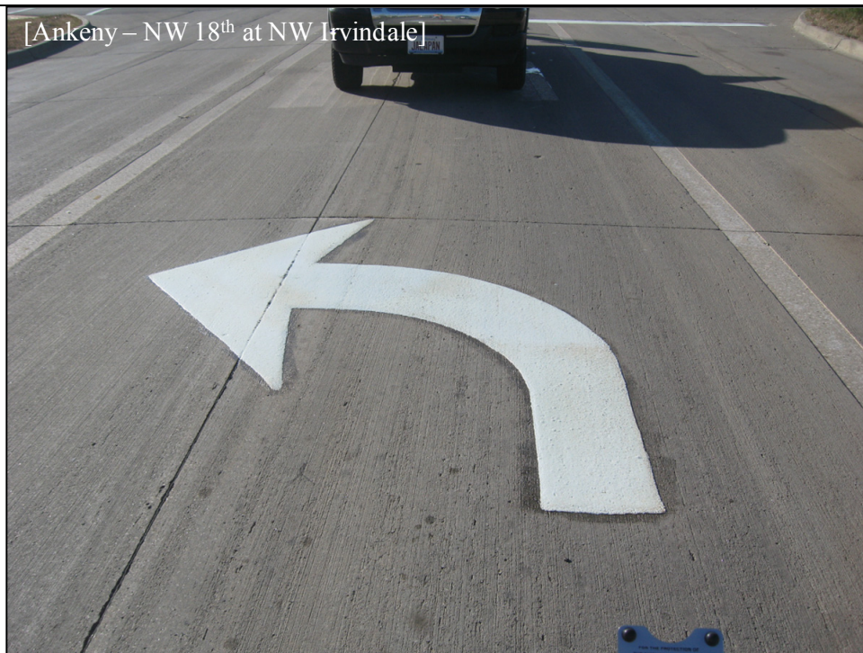
October 2008 – Urban Left Turn Arrow Installation ( R_L=429 ), on concrete.
