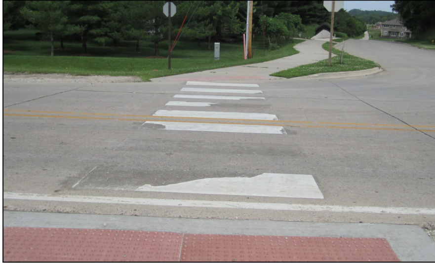
Figure 55. Polk City crosswalk (snow plow damage)
