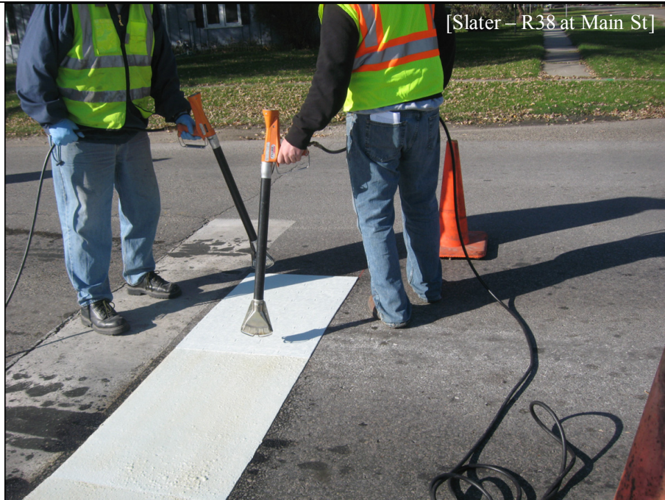
October 2008 – Urban Stop Bar Installation ( R_L=526 ), on asphalt which is rutted within the wheel paths.
