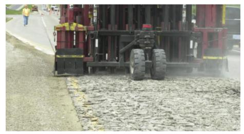
Rubblization using a multiple-head breaker
