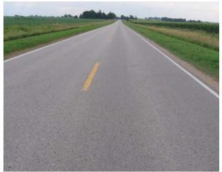
This rubblized PCC pavement overlaid with hot mix asphalt exhibited no cracking.
