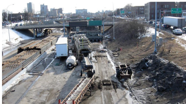
Figure 7.3. Well-implemented on-site material crushing program in urban area
