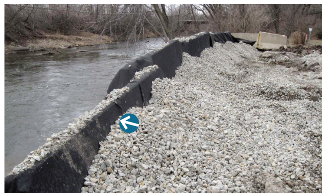
Figure 7.9. Perimeter control at waterway near demolition and concrete crushing operations with RCA filter berm on inside of geotextile-wrapped Jersey barrier
