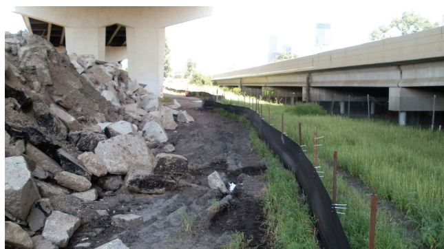
Figure 7.4. Demolished material stockpiled beneath bridge prior to crushing with silt fence and vegetative buffer used
