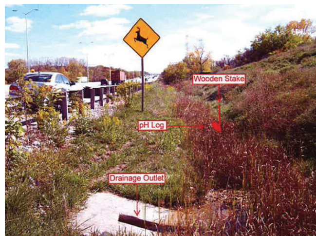
Figure 7.11. Localized mitigation of high-pH leachate from drain near receiving waters using pH log and bioswale
