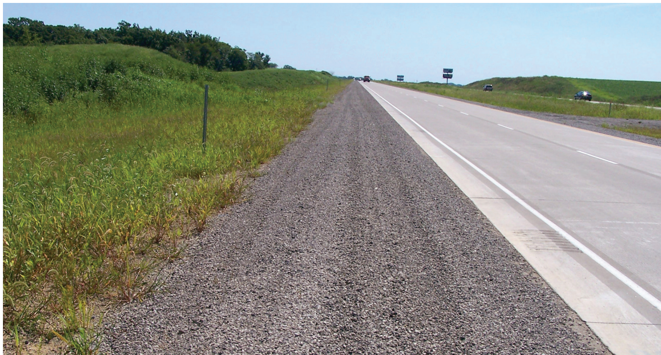
Figure 5.1. RCA aggregate shoulder (50% blend with natural aggregate) on US 34 east of Fairfield, Iowa
