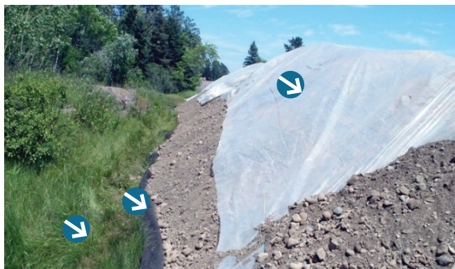
Figure 7.10. RCA stockpile tarped with plastic and bounded by perimeter berm of wrapped RCA
