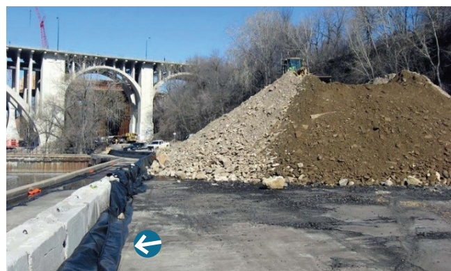
Figure 7.8. High-performance perimeter control using concrete blocks wrapped in geotextile fabric
