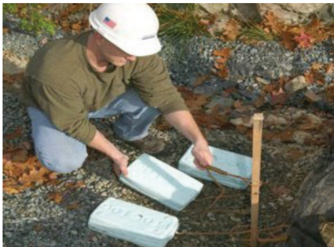
Figure 7.12. Floc Bloc tied to wooden stake in outflow path
