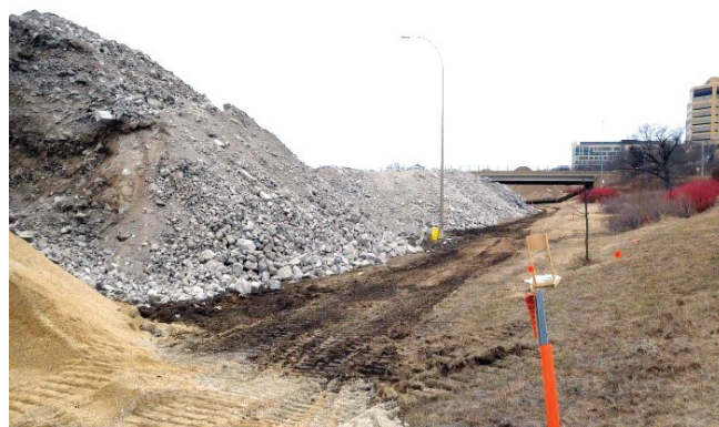
Figure 7.7. Concrete stockpiles set inside of roadway depression with stormwater inlets taken offline
