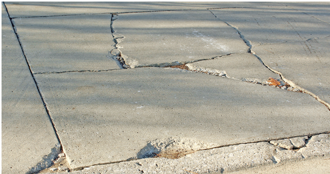
Figure 3-8. Shattered slab
