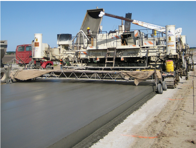
Figure 8-5. Trackline of slipform paving machine
