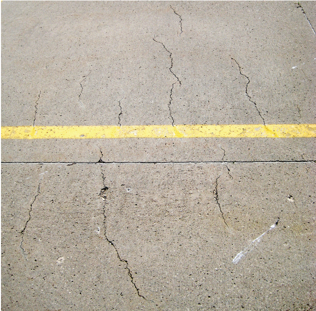
Figure 6-26. Plastic shrinkage cracks
