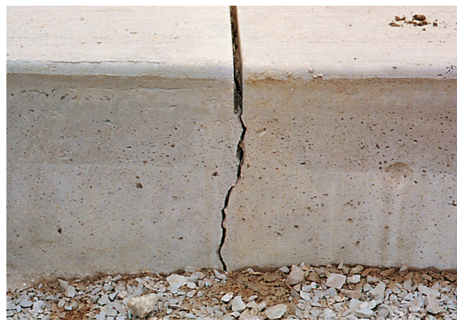
Figure 6-23. A saw cut that has cracked through as planned
