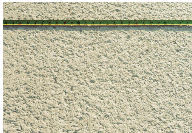
Figure 8-30. Typical scaling of concrete pavement due to rain, resulting in nondurable paste surface
