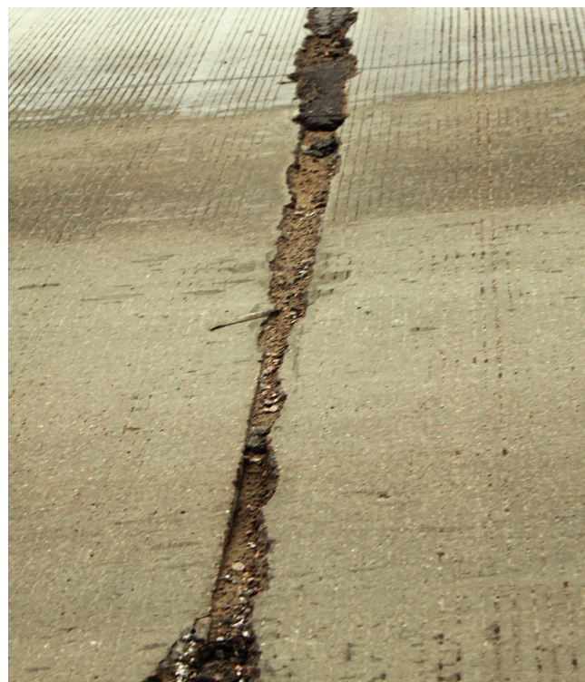
Figure 6-34. Joint damage
