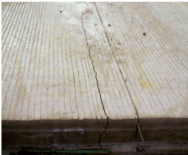
Figure 6-24. This joint was cut too late, resulting in random transverse cracking
