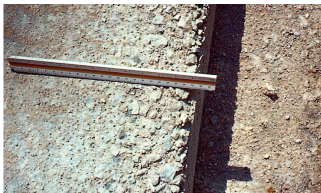
Figure 8-31. Edge erosion of freshly placed slab due to rain
