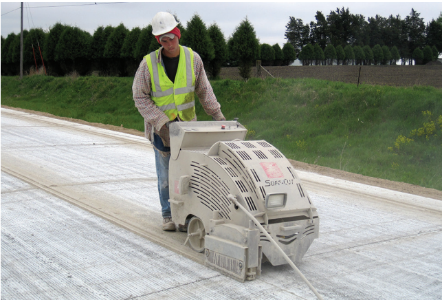
c) Early-entry, walk-behind dry saw
