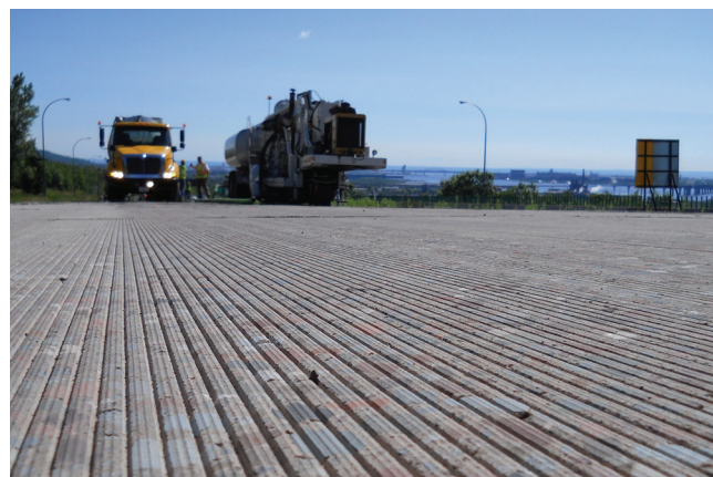
Figure 8-22. Next-generation concrete surface (NGCS)
