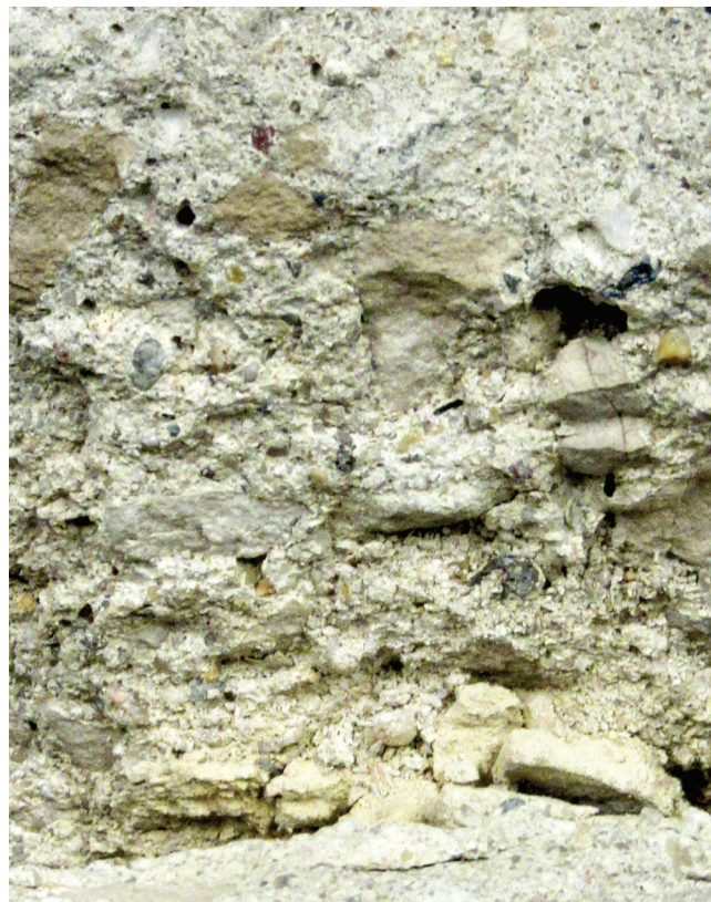
Figure 6-33. Joint damage showing flakes
