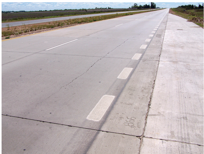
Figure 6-29. Random longitudinal crack
