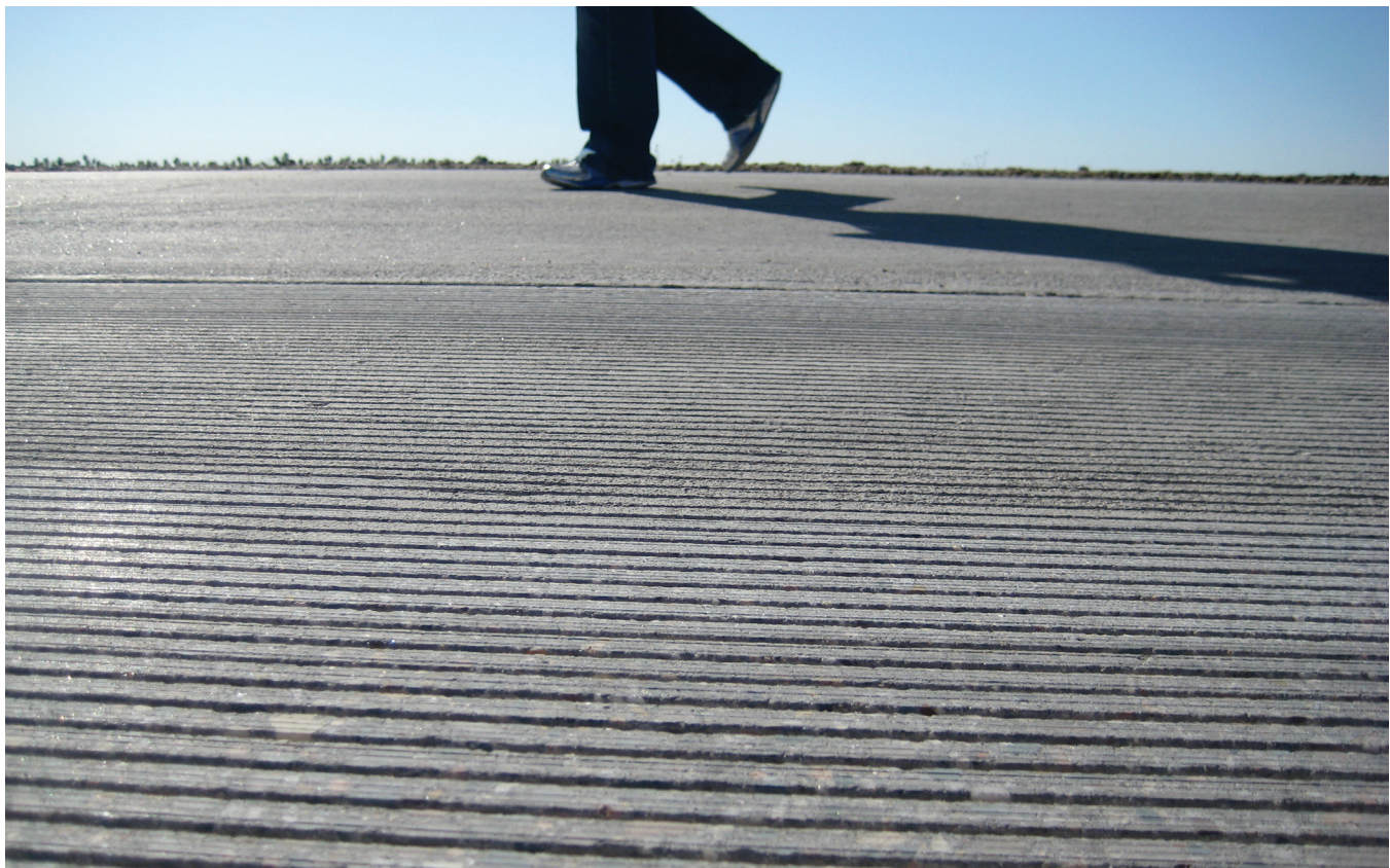
Figure 3-11. Next-generation concrete surface (NGCS)
