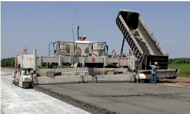
ACPA, used with permission Figure 8-11. A belt placer/spreader ensures a consistent amount of concrete in front of the paver
