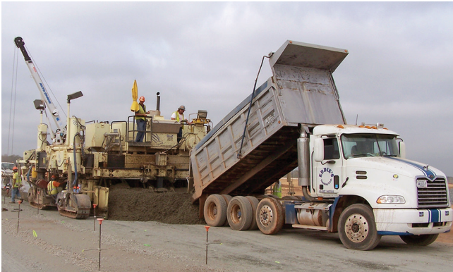
ACPA, used with permission Figure 8-10. Depositing concrete in front of the paving machine
