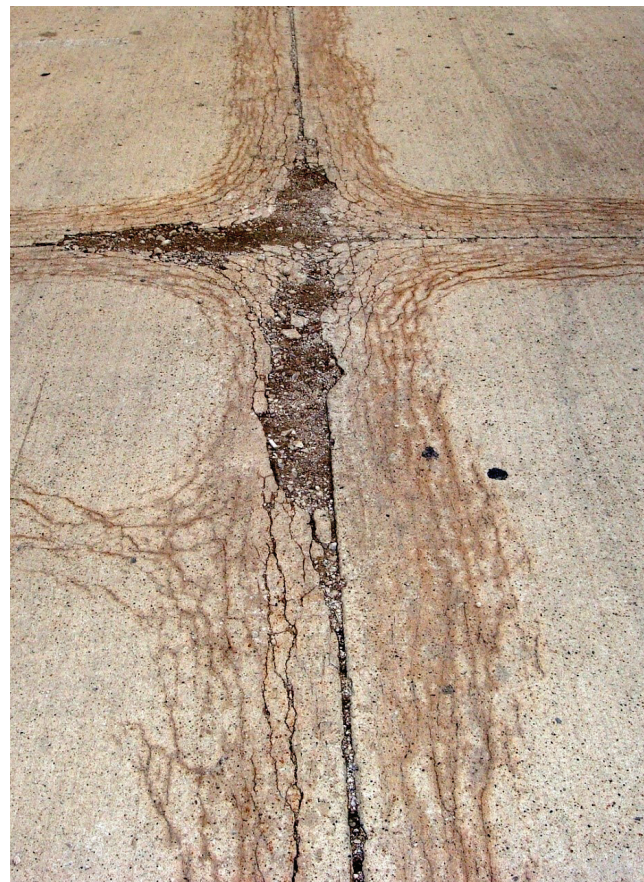
Figure 6-36. D-cracking
