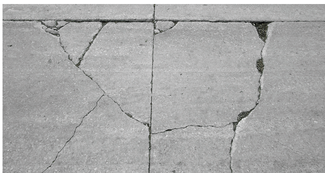
Figure 3-5. Corner cracking in jointed concrete pavement
