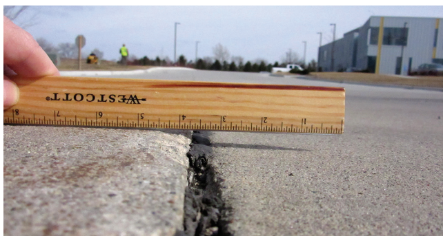
Figure 3-9. Faulting
