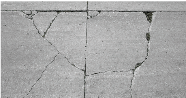
Figure 6-30. Corner break
