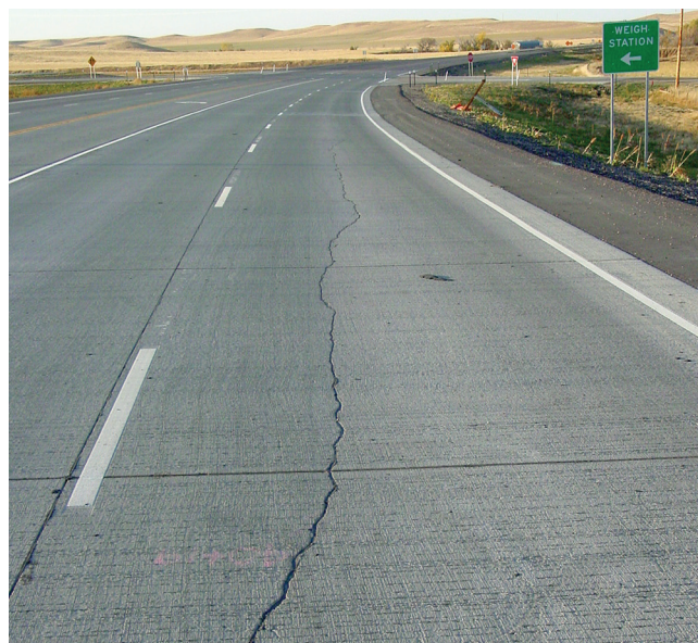
Figure 3-7. Structural longitudinal crack
