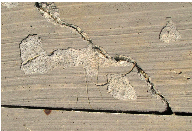
Figure 6-35. Scaling
