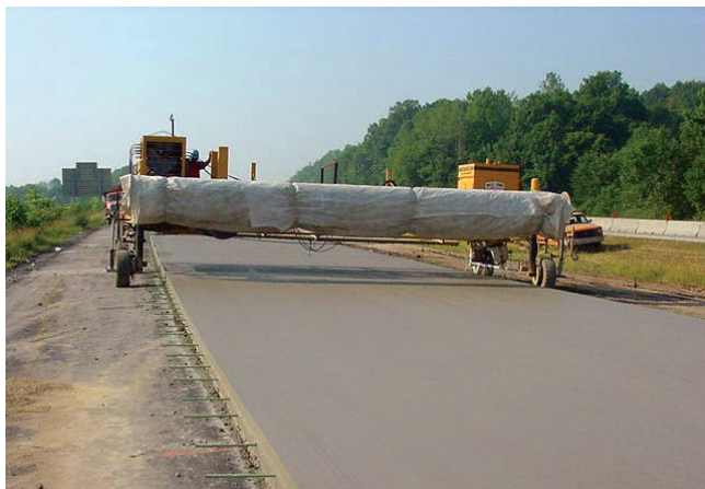
Figure 8-29. Plastic sheeting ready for placement to protect the fresh surface from rain
