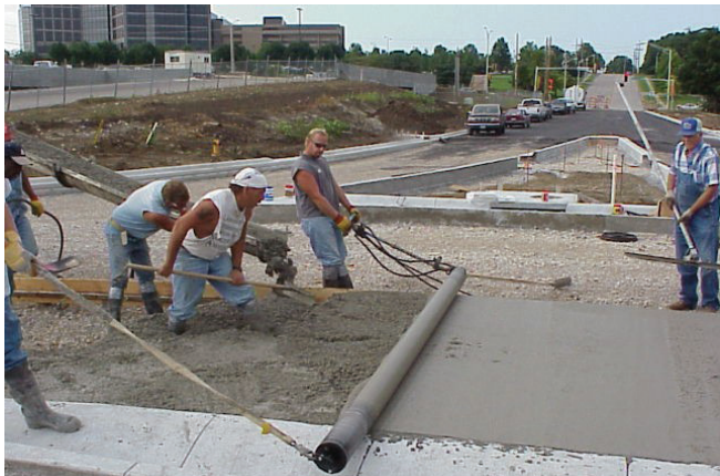
Figure 8-12. A roller screed (single-tube finisher) can be used to strike off the concrete in fixed-form placements
