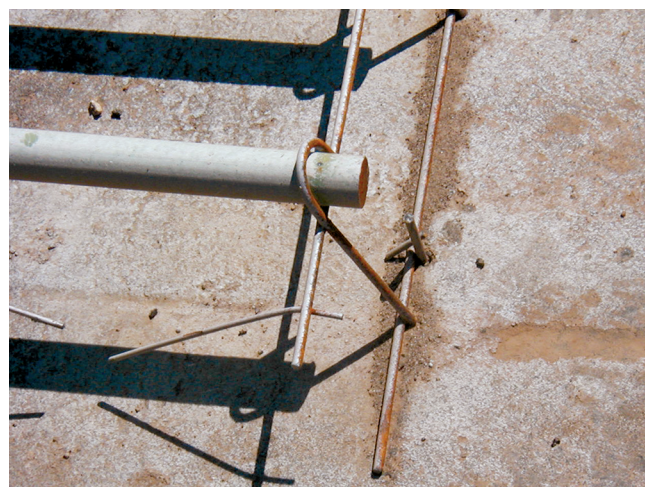
Figure 8-19. Staking or pinning dowel bar cages
