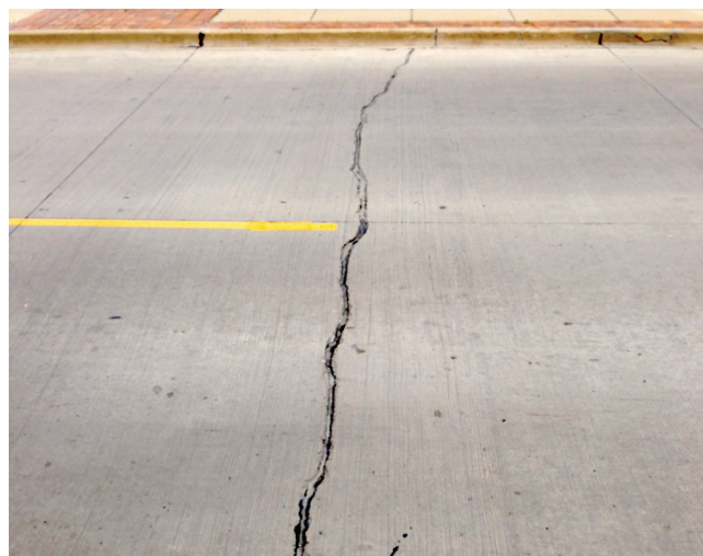
Figure 3-6. Structural transverse crack
