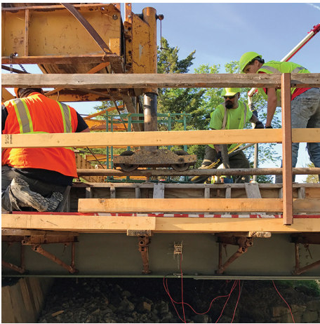
Maple Bridge instrumentation and temporary timber blocking and diagonal cross-bars for the east (left) and west (right) spans during the braced deck pour
