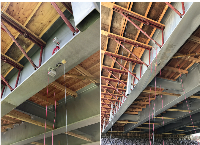
Maple Bridge instrumentation and temporary timber blocking and diagonal cross-bars for the east (left) and west (right) spans during the braced deck pour
