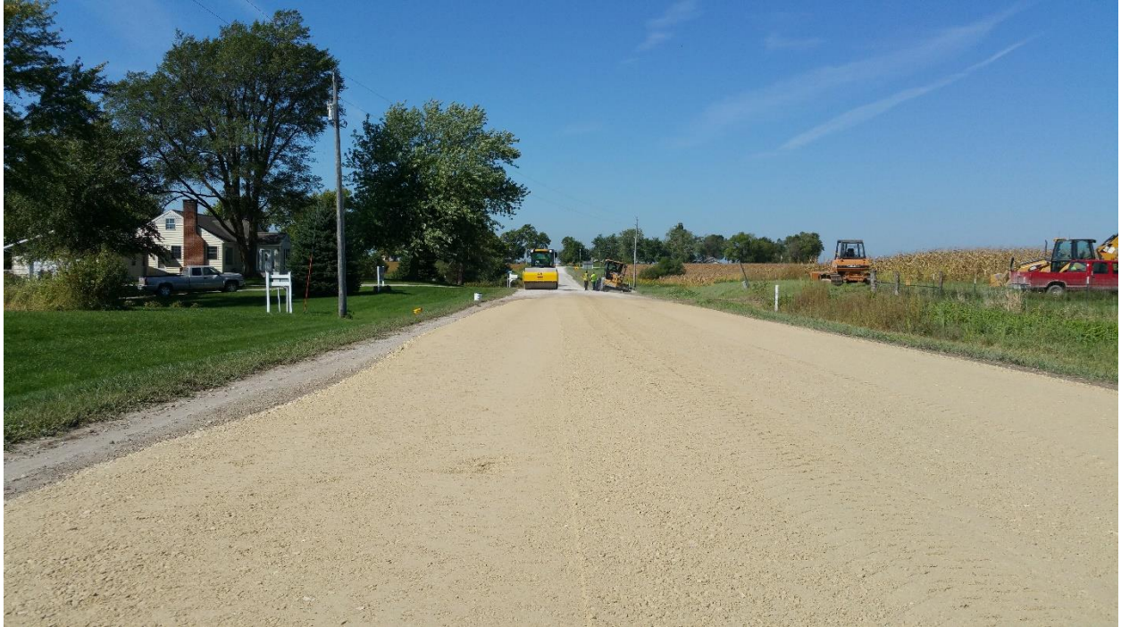
Figure A.10. Second section during drum roller compaction
