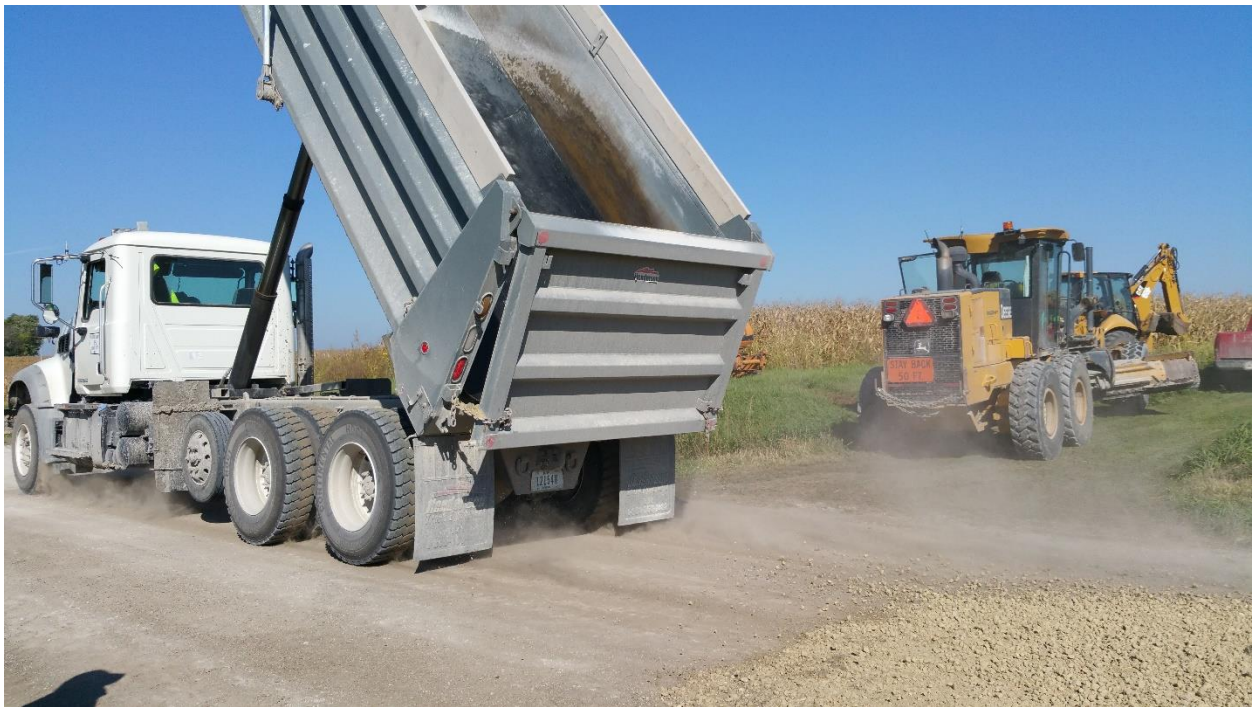
Figure A.7. OFD Class A materials dumped on the second section
