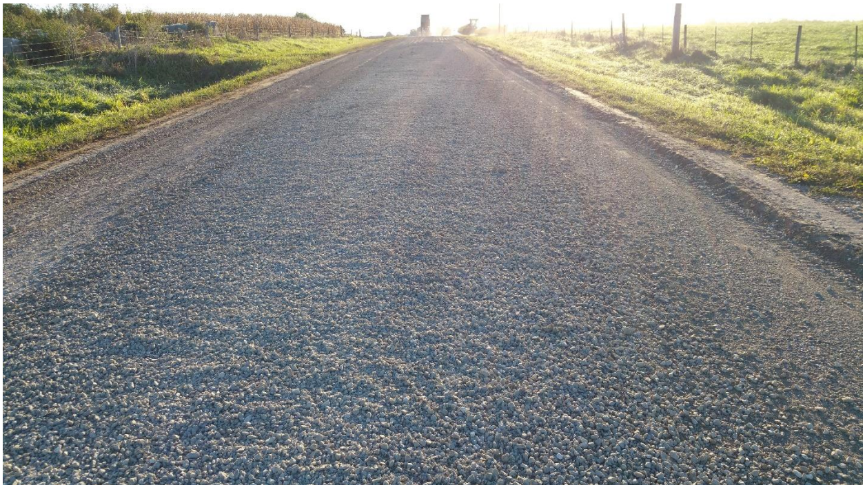
Figure A.23. Wheel compacted surface of 70% BFL Class A + 30% LCF Clean
