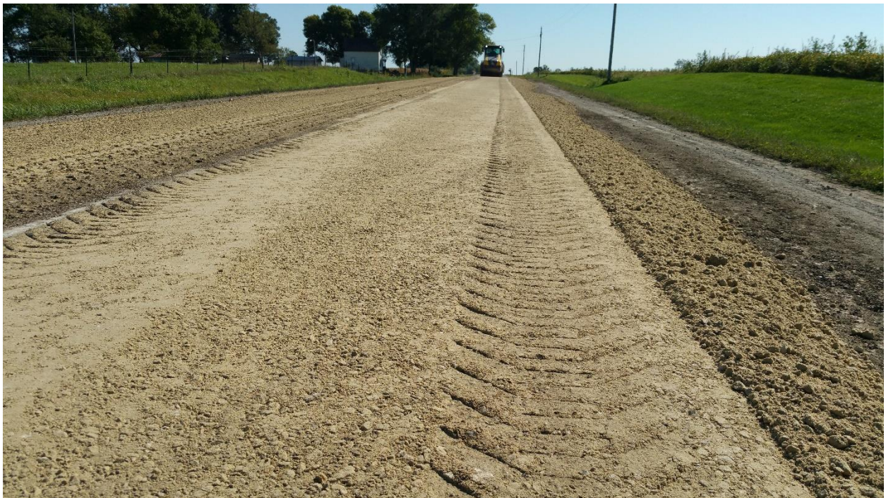
Figure A.9. Wheel compacted OFD Class A materials in second section
