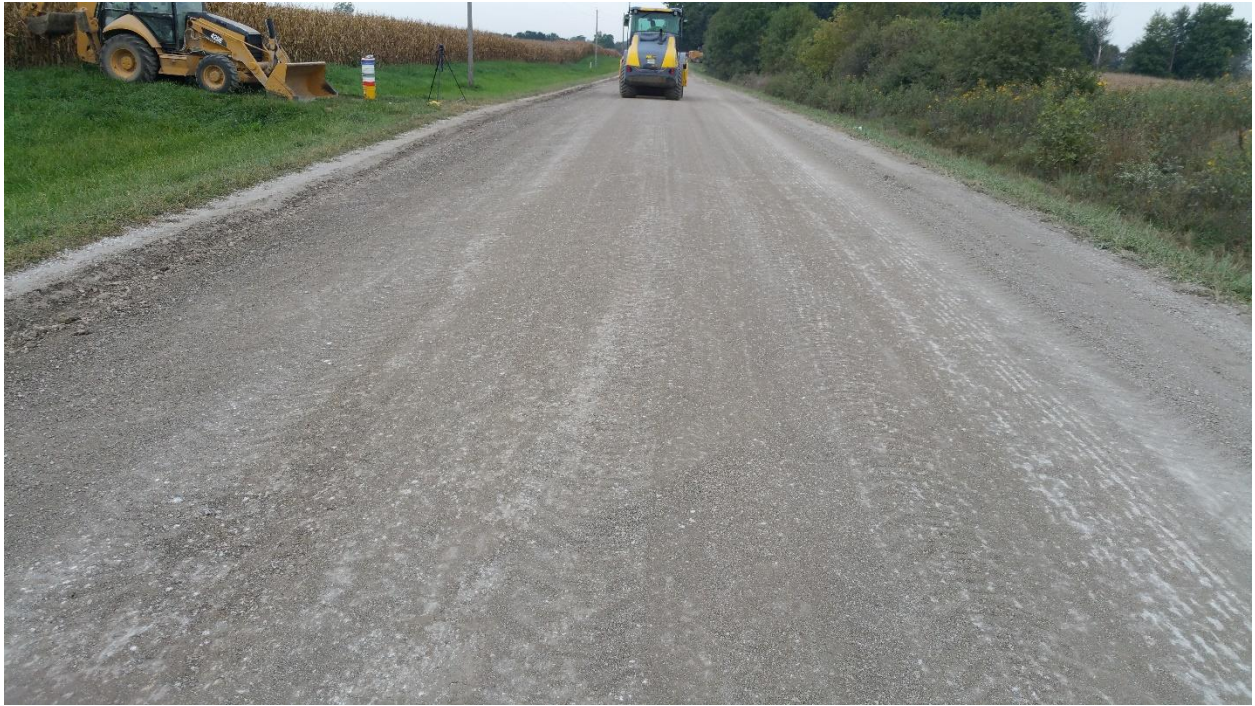
Figure A.16. Scraped surface of the fifth section before construction during drum roller compaction
