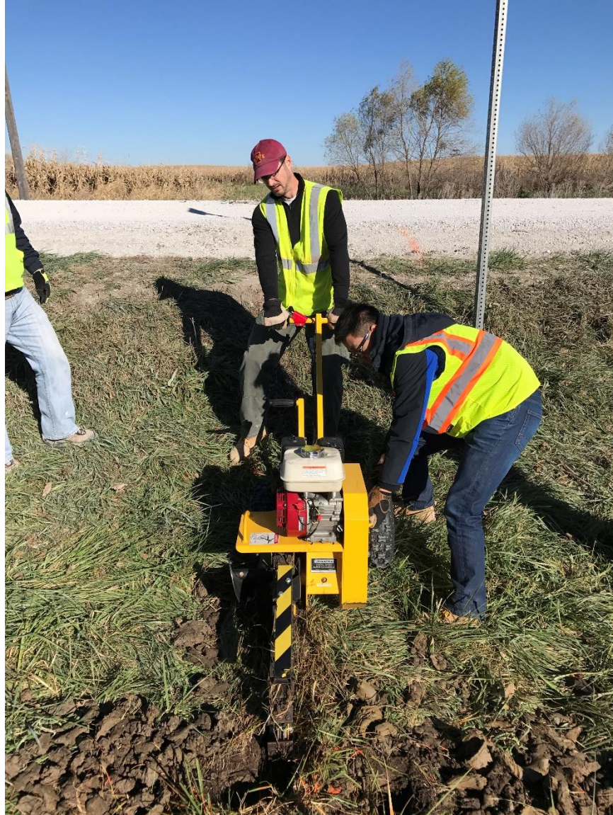
Figure E.4. Digging the surface for the thermocouple installation
