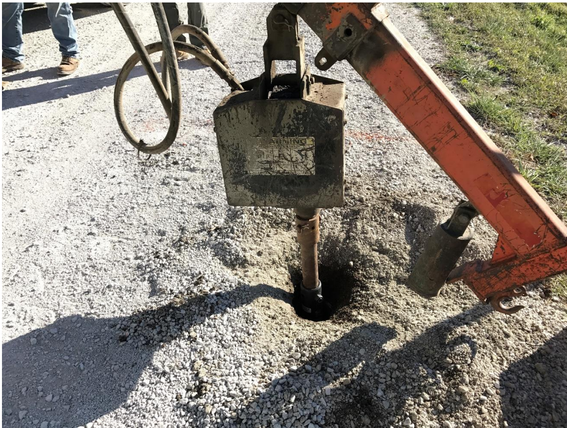
Figure E.1. Borehole digging with auger at center and shoulder of the road
