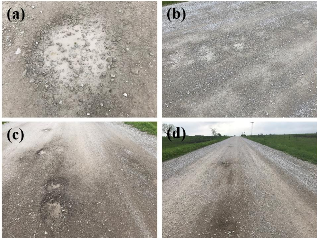
Figure 49. Distress types on surface materials: (a) big pothole in middle of BFL Class A, (b) severe rutting in 80% BFL Class A + 20% BFL Clean, (c) scattered potholes in 70% BFL Class A + 30% LCF Clean, and (d) material movement 70% BFL Class A + 30% CRG
