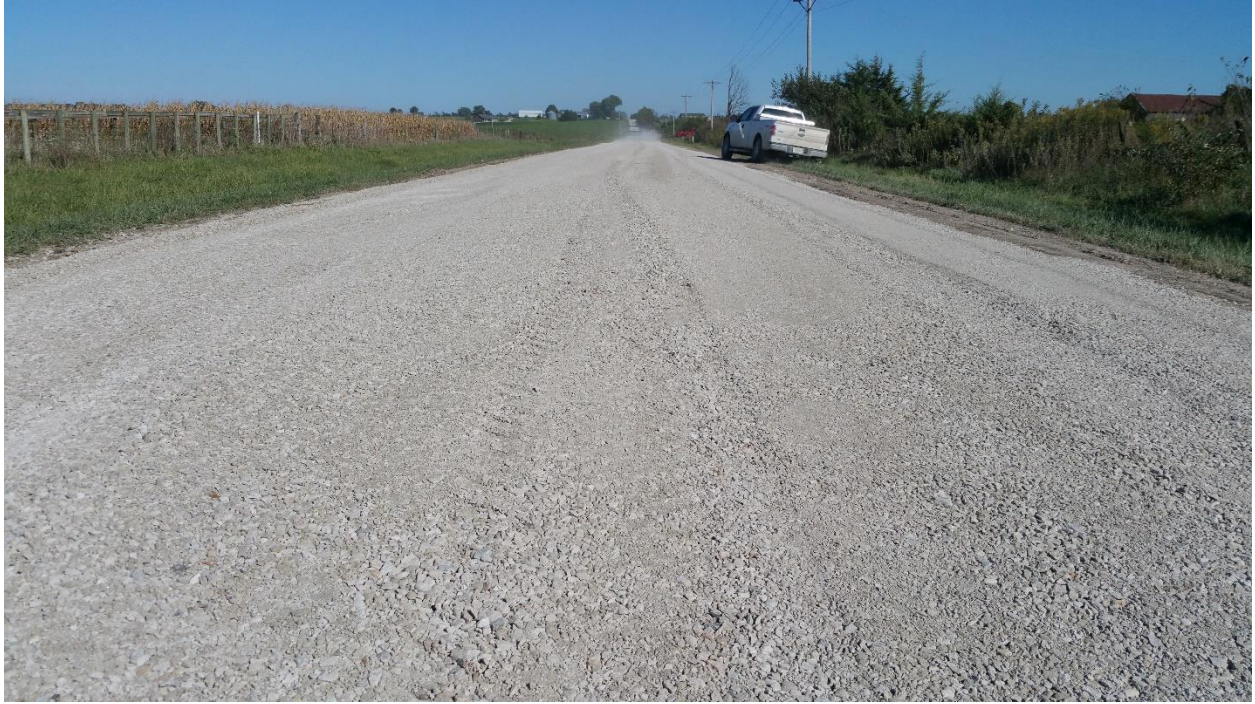
Figure A.28. Shaped and compacted surface of 70% BFL Class A + 30% CRG Clean
