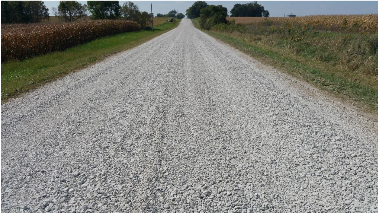
Figure A.14. The mixture of the BFL Class A and Clean on the fourth section
