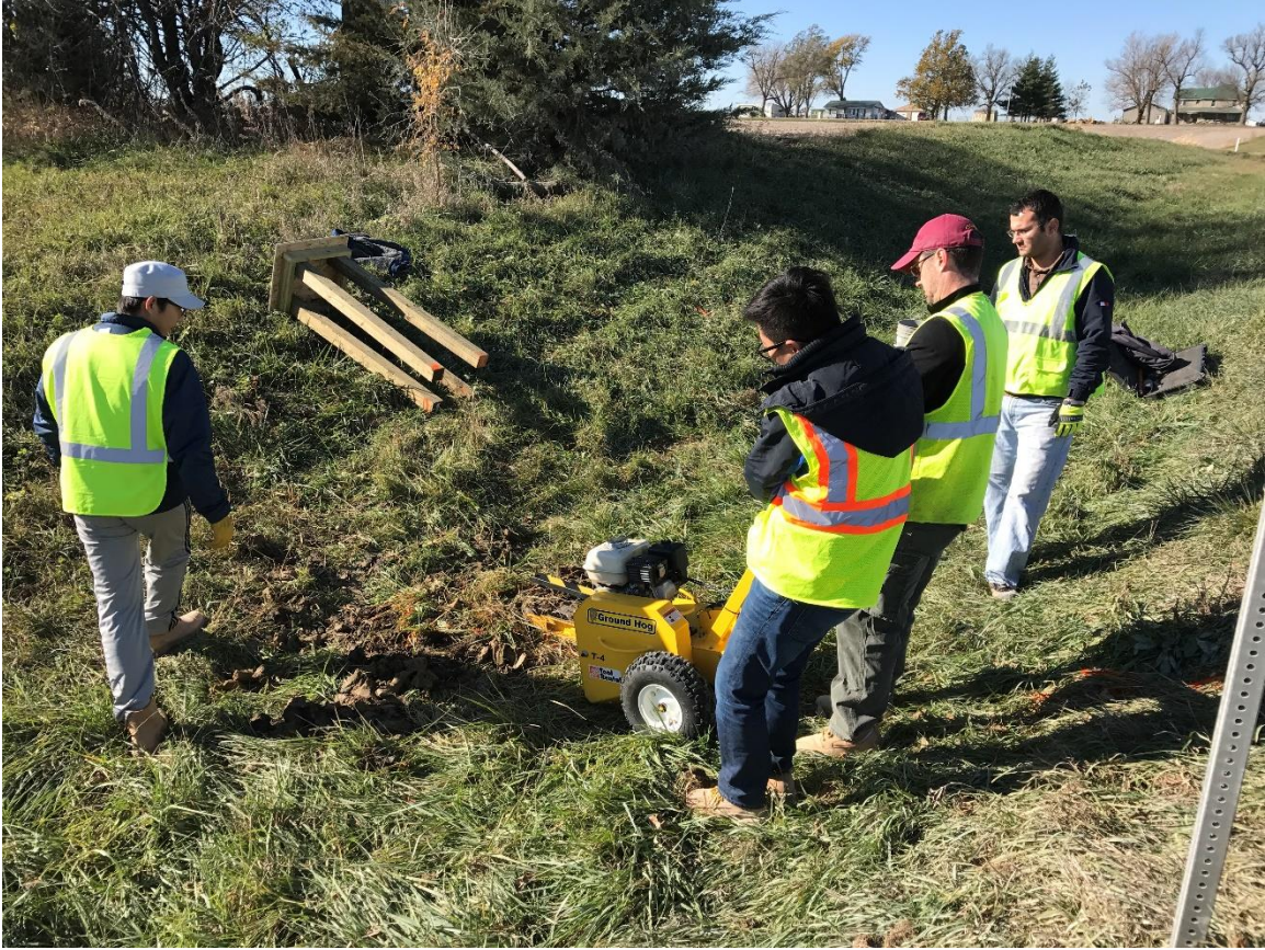
Figure E.3. Digging the thermocouple path with auger
