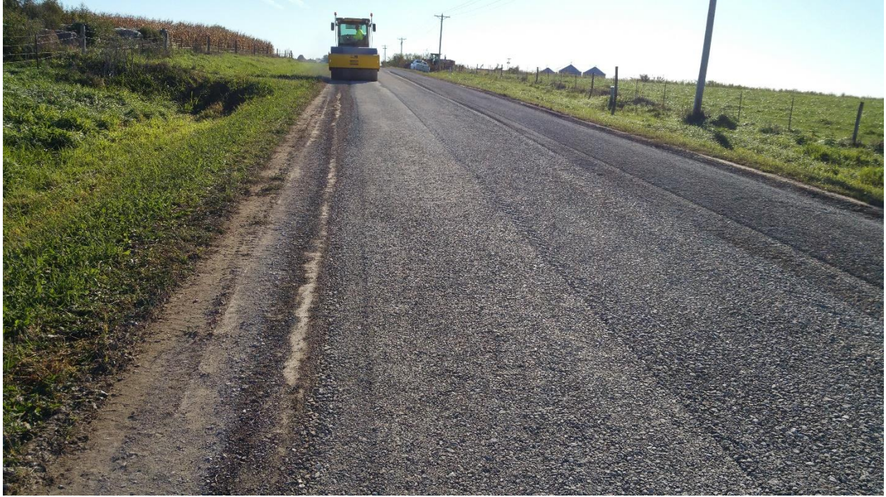
Figure A.22. 70% BFL Class A + 30% LCF Clean under compaction
