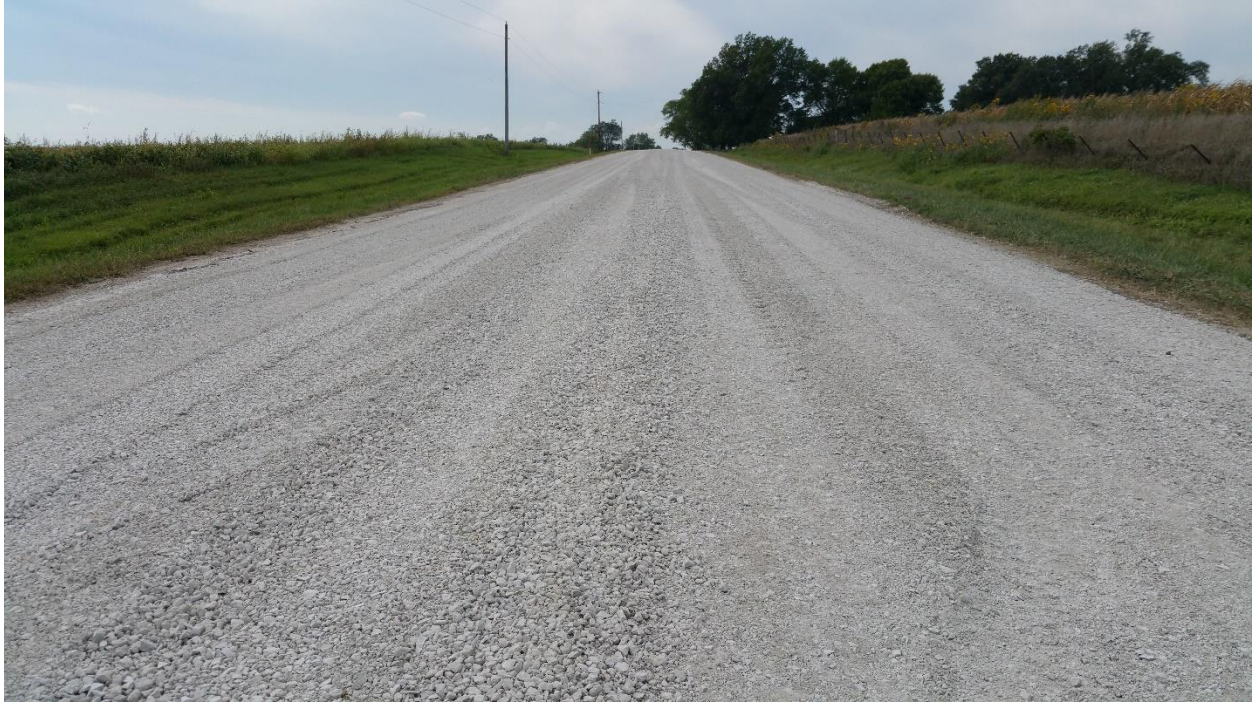
Figure A.12. Wheel compacted surface of the third section
