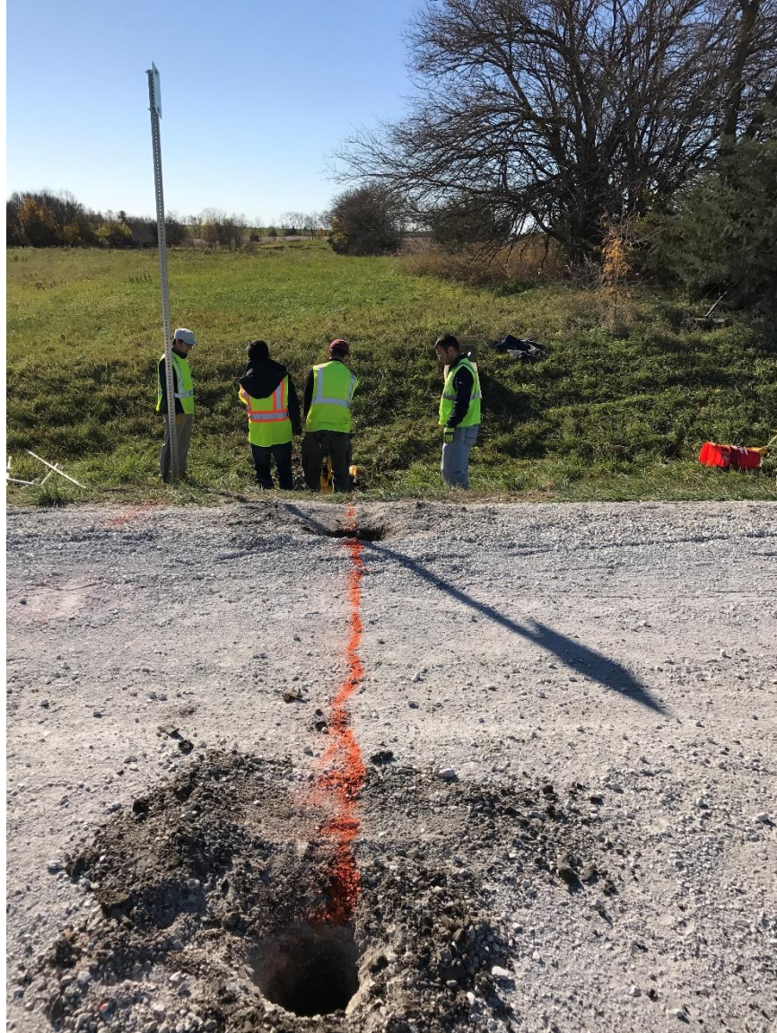
Figure E.2. Painting the thermocouple path
