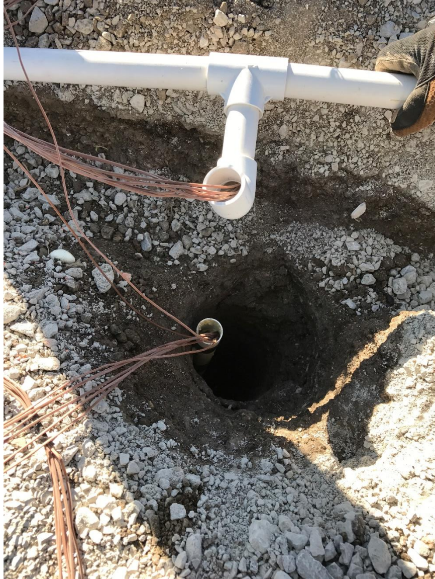
Figure E.5. Thermocouples at PVC tubes
