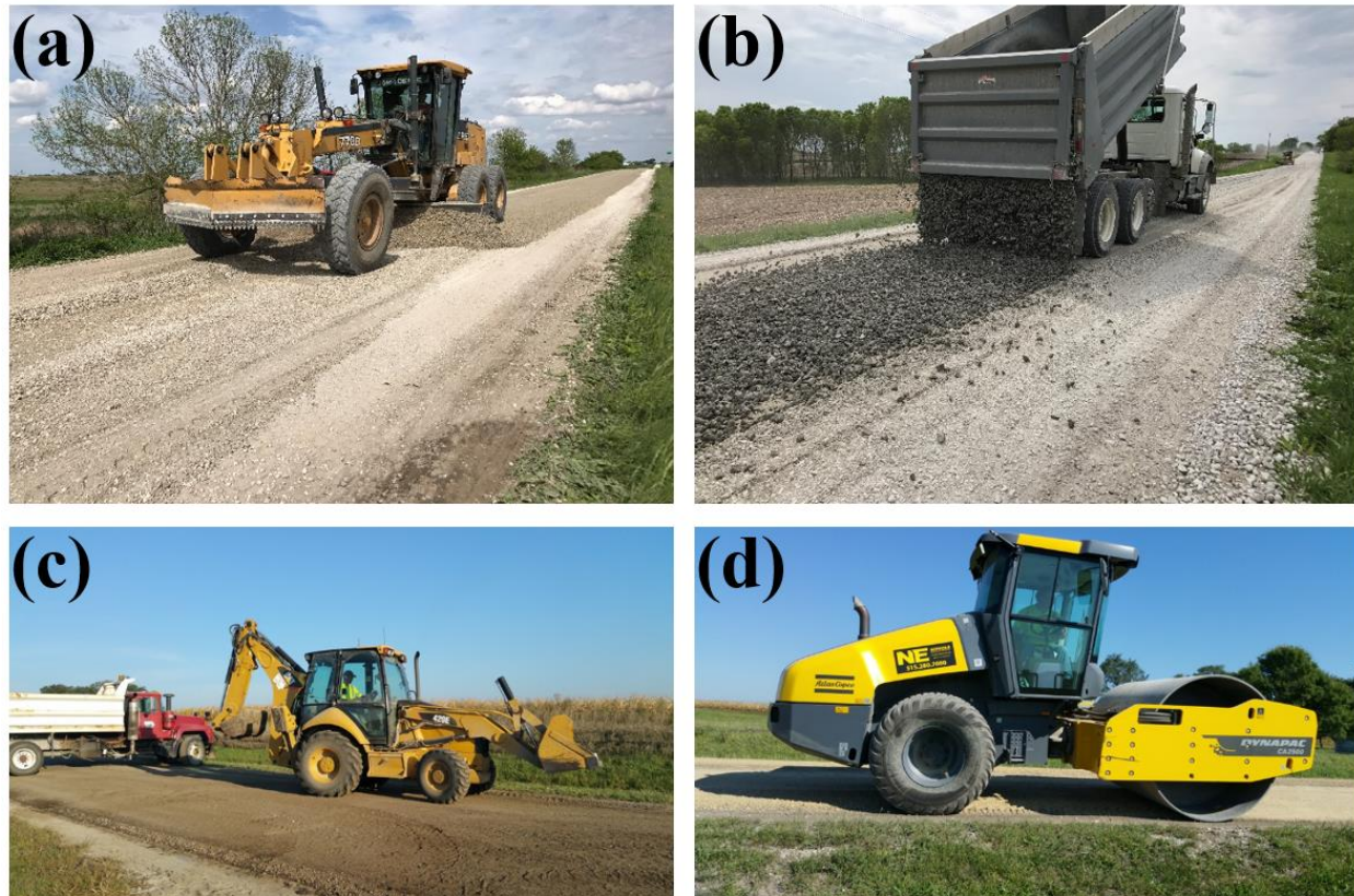
Figure 50. Equipment used: (a) motor grader for blading, (b) dump trucks, (c) loader for collection the existing chip seal layer, and (d) vibratory roller for compaction
