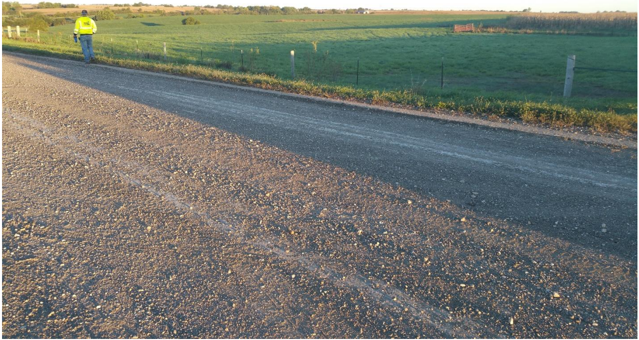
Figure A.24. Prepared surface of 70% BFL Class A + 30% LCF Clean
