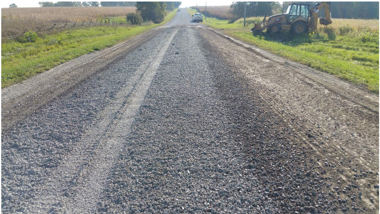
Figure A.11. BFL Class A materials on the third section
