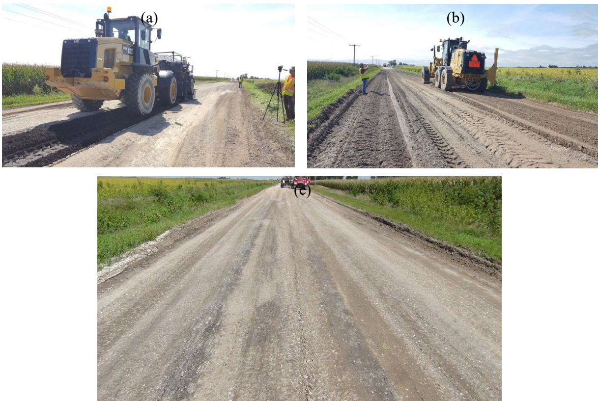
Figure 40. Construction of BASE ONE section in Hamilton County: (a) incorporating stabilizer into surface course with RoadHog, (b) blading with motor grader, and (c) finished surface after final compaction and blading
