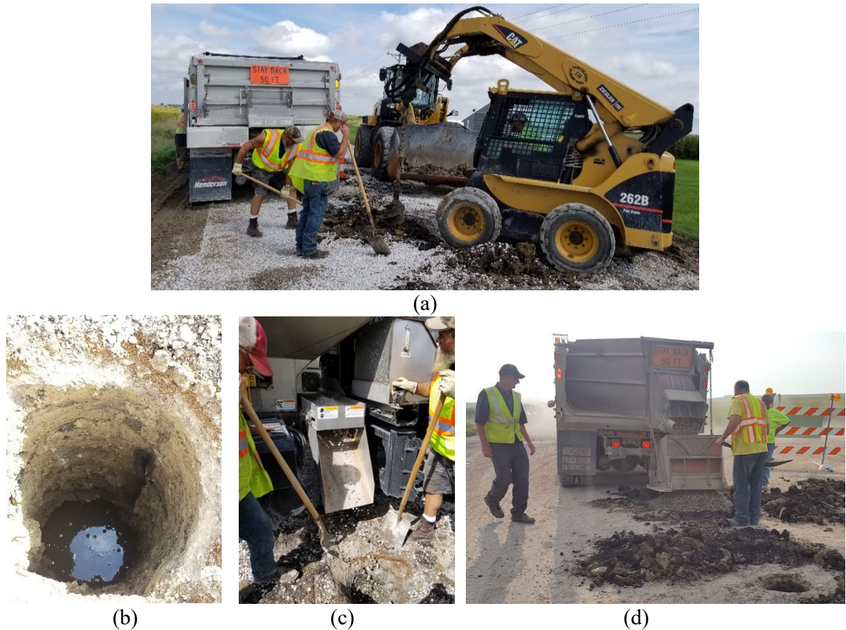
Figure 22. Aggregate columns installation: (a) drilling hole with skid steer-mounted power auger, (b) completed hole, (c) backfilling hole with clean aggregate using side chute, and (d) backfilling with hopper
