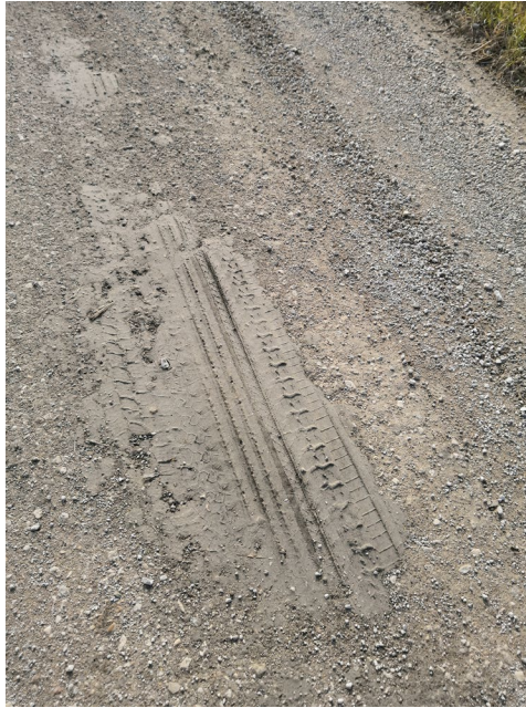
Figure 129. Clay on the surface in Hamilton County Claycrete section
