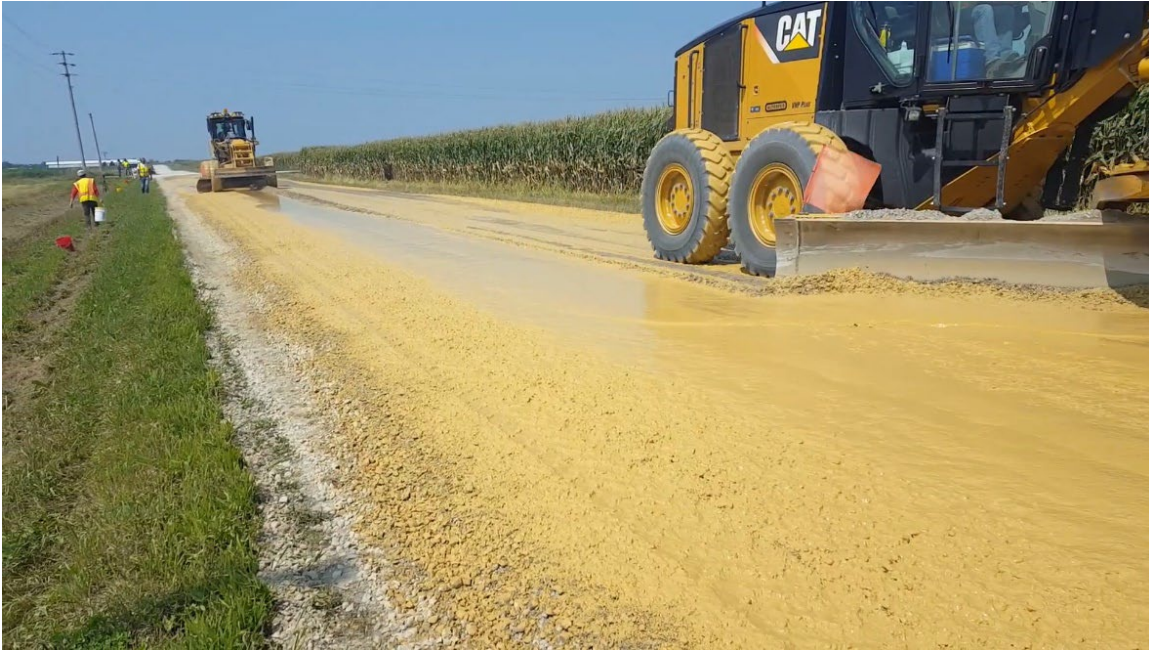
Figure 26. Consistency of clay slurry and aggregate at beginning of blade mixing process in Washington County
