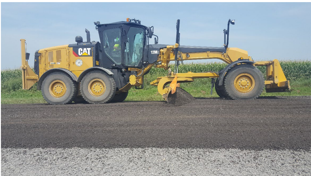
Figure 30. Blading Phoenix slag in Howard County
