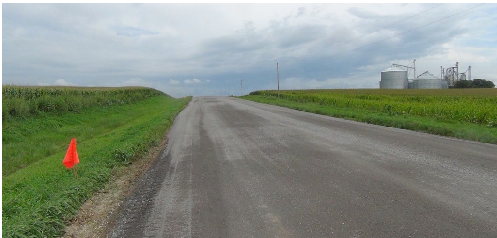
Figure 34. 4 in. completed surface of Harsco slag section in Howard County
