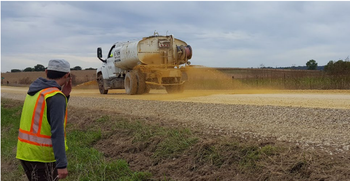
Figure 25. Tanker used for spreading clay slurry in Cherokee County
