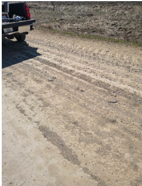
Figure 128. Rutting in Howard County OGCS section during spring 2020
