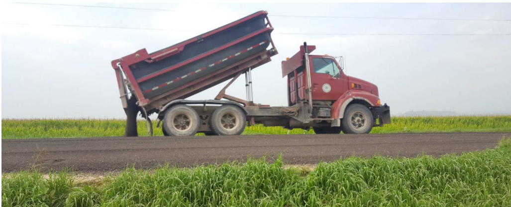
Figure 33. Dumping Harsco slag over the subgrade in Howard County
