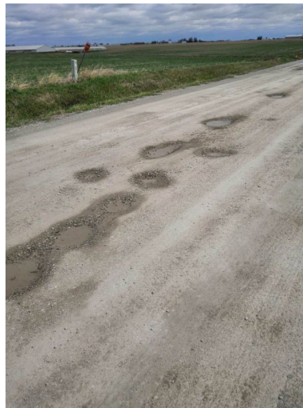
Figure 130. Potholes in control section in Washington County during spring 2020
