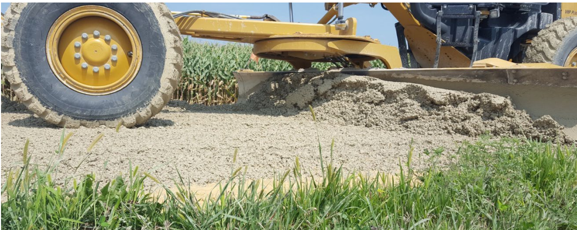
Figure 28. Consistency of clay slurry and aggregate near the end of blade mixing process in Washington County
