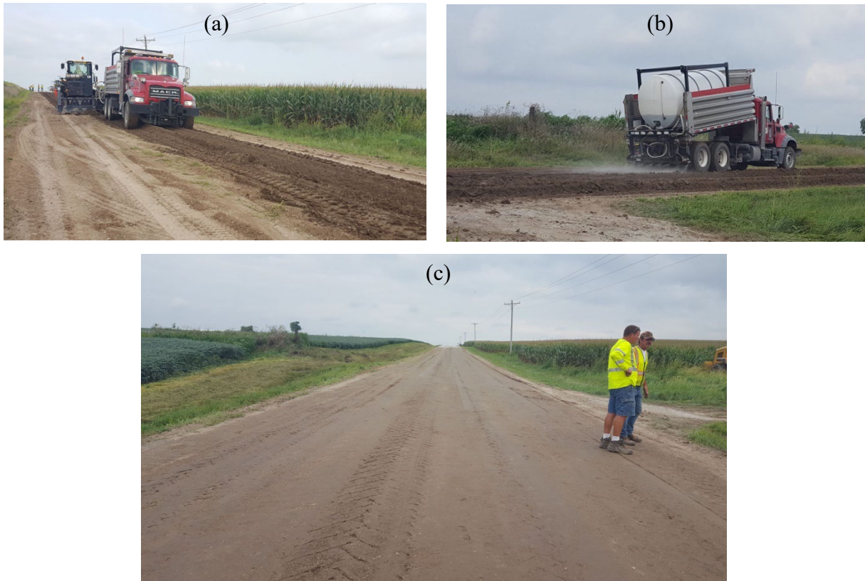
Figure 41. Construction of EMC SQUARED section in Washington County: (a) incorporating stabilizer into the subgrade with RoadHog, (b) spraying stabilizer over aggregate surface, and (c) finished surface after mixing, blading, and final compaction
