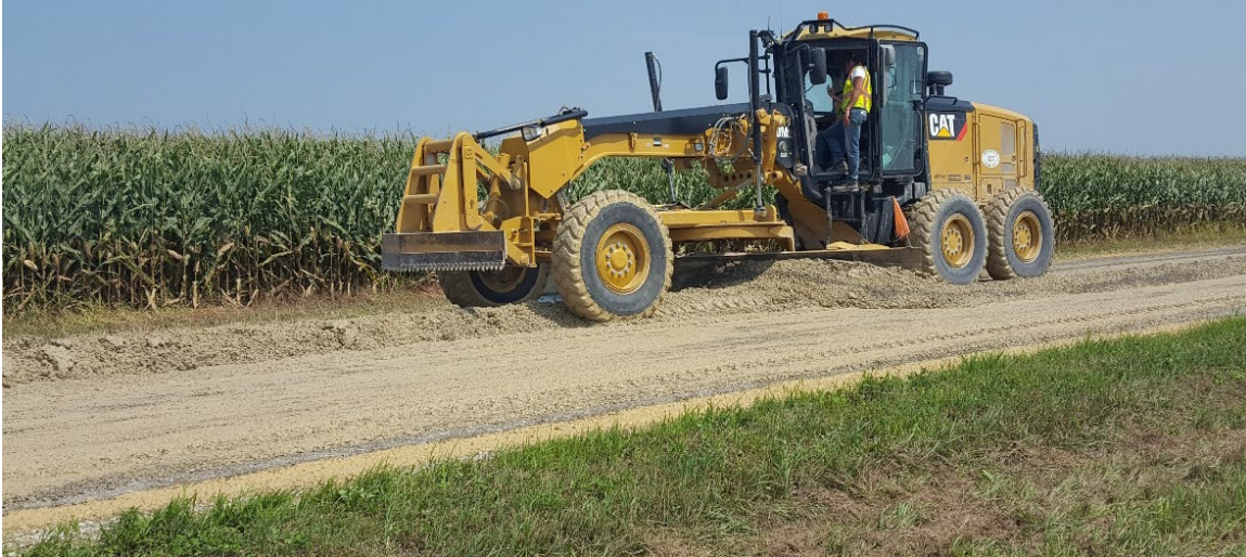
Figure 27. Clay slurry and aggregate near the end of the blade mixing process in Washington County
