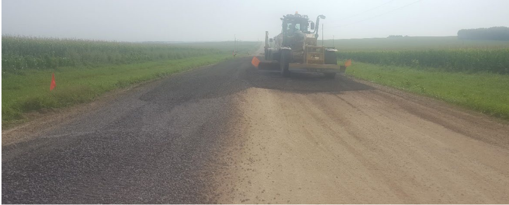
Figure 29. Spreading Phoenix slag over the subgrade in Howard County
