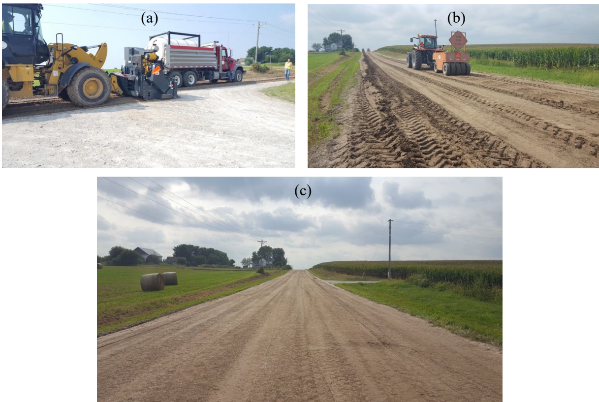
Figure 39. Construction of BASE ONE section in Washington County: (a) incorporating stabilizer into surface course with RoadHog, (b) compacting with rubber tire roller, and (c) finished surface after final compaction and blading
