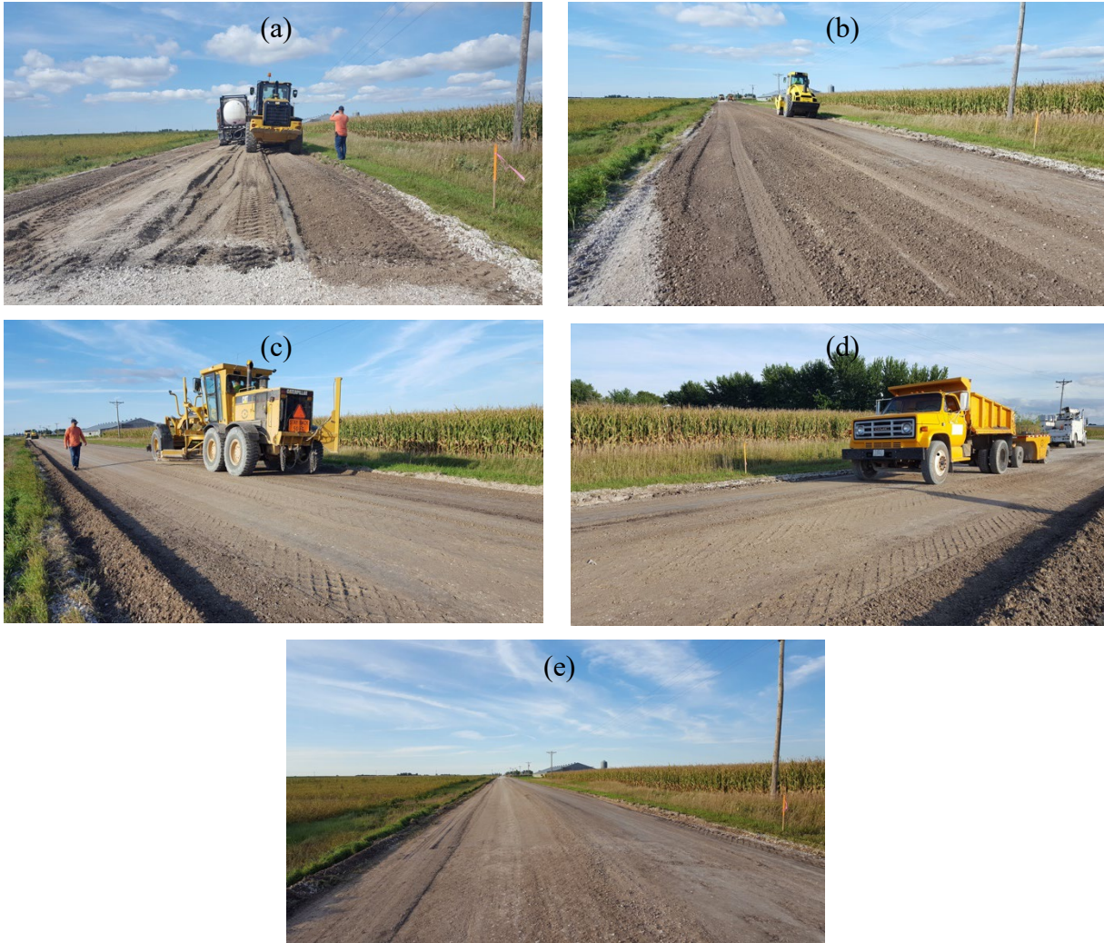
Figure 44. Construction of Claycrete section in Hamilton County: (a) milling stabilizer into aggregates and subgrade, (b) compacting with smooth drum vibratory roller, (c) blading surface, (d) compacting with rubber tire roller, and (e) finished surface
