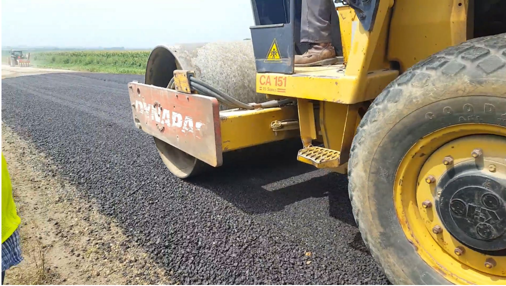
Figure 32. Compacting Phoenix slag with smooth drum vibratory roller in Howard County
