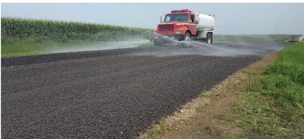
Figure 31. Spraying compaction water over Phoenix slag in Howard County
