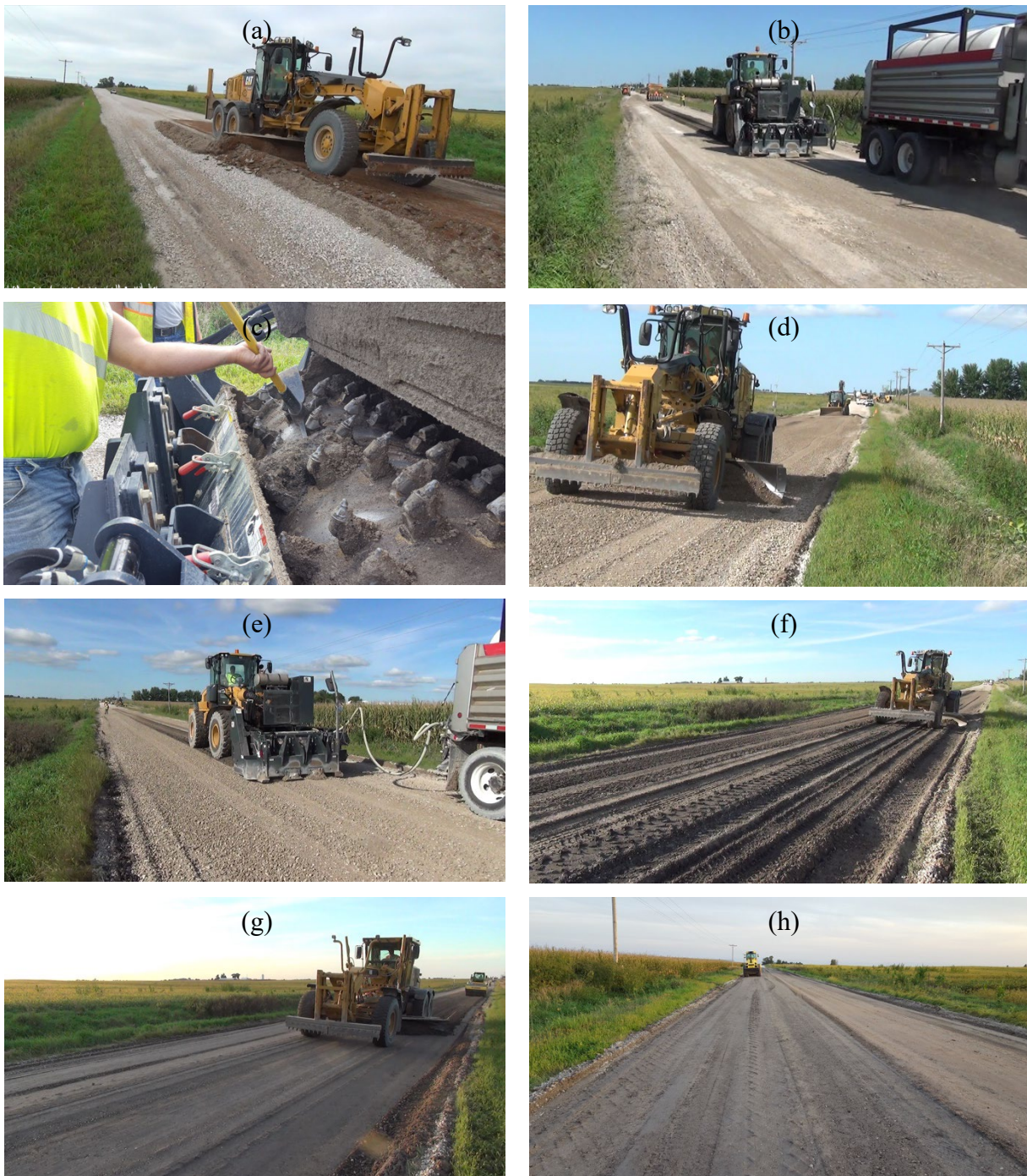
Figure 42. Construction of EMC SQUARED section in Hamilton County: (a) windrowing and removing existing aggregate, (b) stabilizing the subgrade, (c) removing large cobbles from RoadHog, (d) replacing aggregate course, (e) stabilizing aggregate course, (f) leveling surface, (g) blading and compacting surface, and (h) continued compaction
