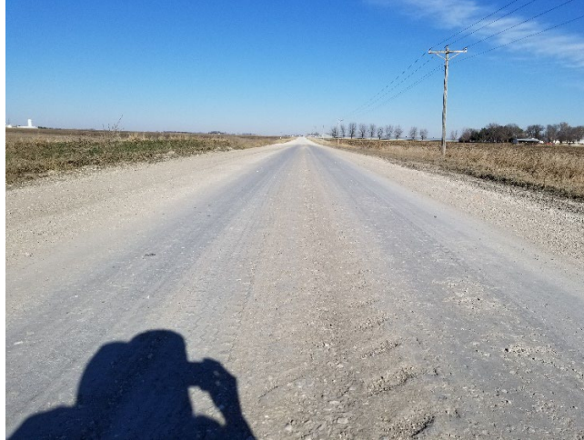
Figure 127. Rutting in EMC SQUARED section in Hamilton County during spring 2019
