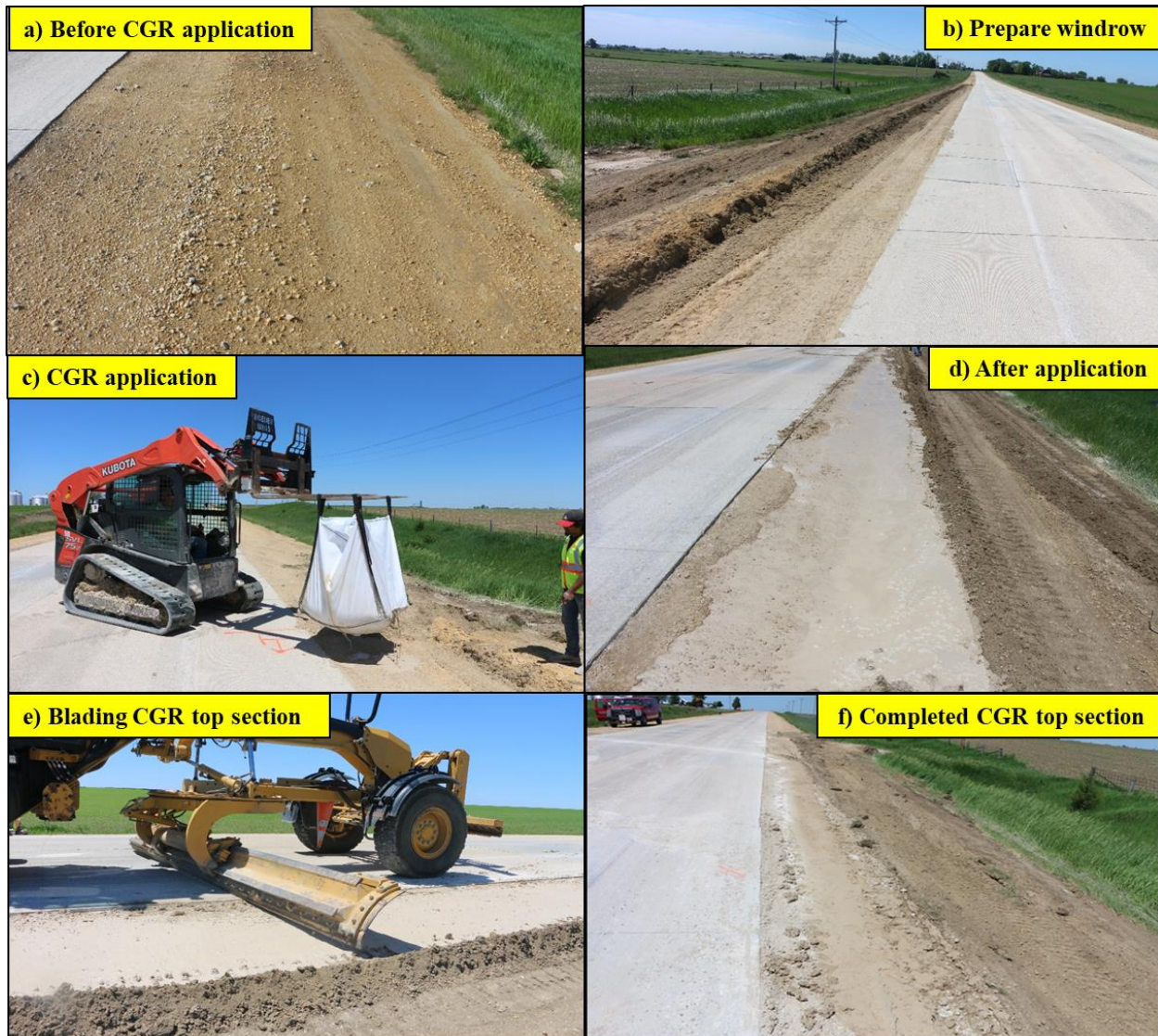
Figure 61. Construction of CGR Top section in Clinton County: (a) section appearance before CGR application, (b) creating windrow, (c) dumping CGR, (d) section appearance after CGR application, (e) blading CGR Top section, and (d) completed CGR Top section
