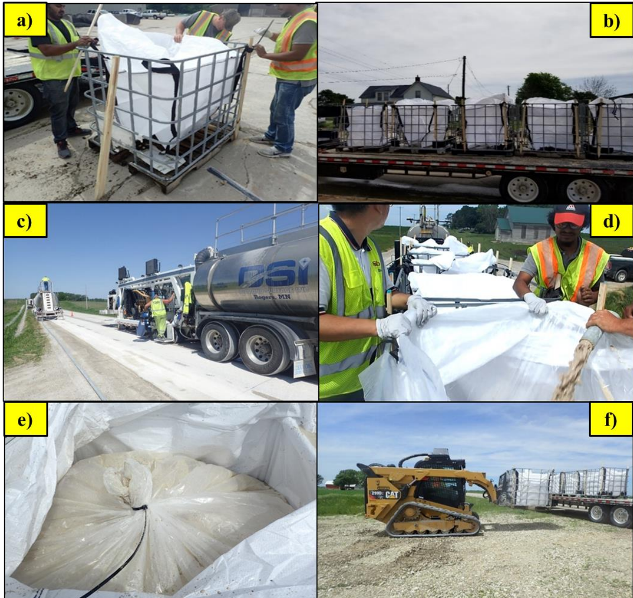
Figure 50. CGR collection at diamond grinding project site in Washington County: (a) preparing the super bags with containment, (b) transporting the super bags to the diamond grinding site, (c) diamond grinding operations, (d) filling the super bags with CGR, (e) securing the bags, and (f) transporting the bags to the construction site
