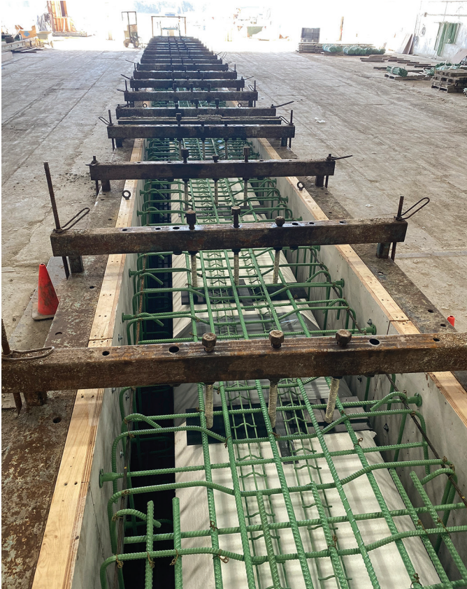
Box girder form with reinforcement in precast concrete plant
