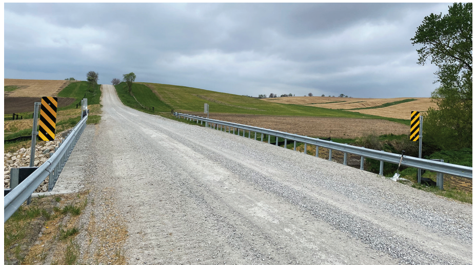
Completed box girder bridge in Washington County, Iowa
