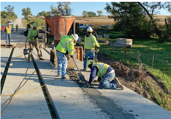
Placement of joint concrete in the field
