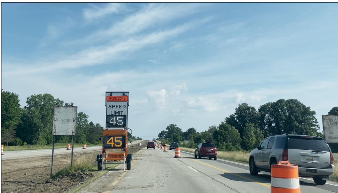
Figure 9. SFT + DSL assembly deployed in a freeway lane closure in Michigan
