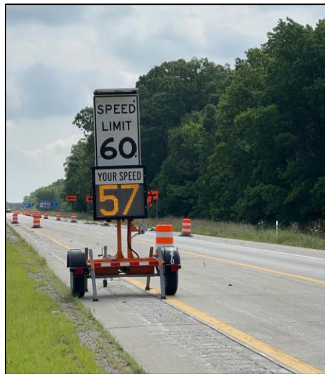
Example speed feedback trailer in a freeway work zone lane closure in Michigan
