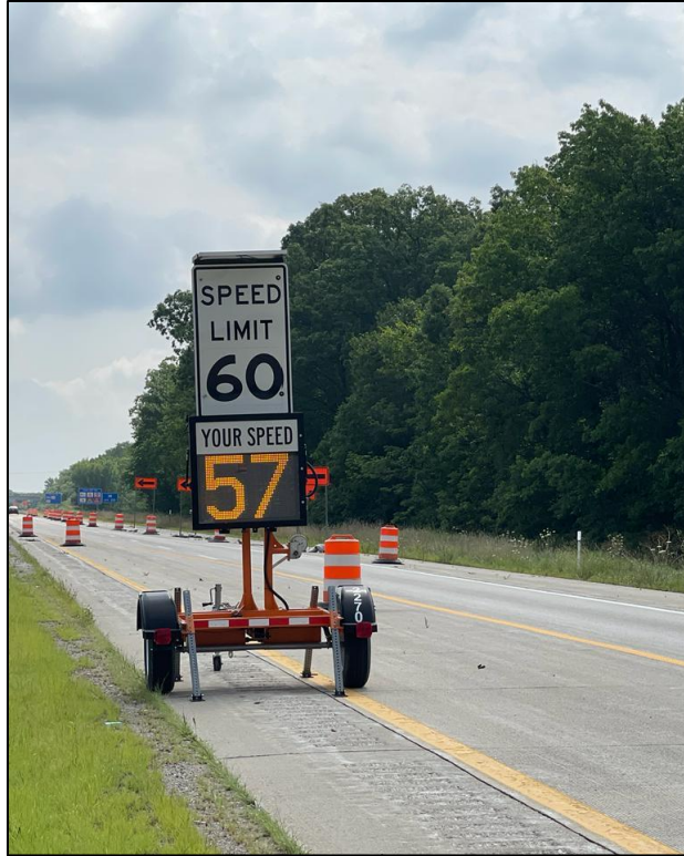
Figure 8. Speed feedback trailer in a freeway work zone lane closure in Michigan
