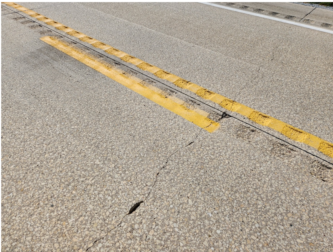
Figure 36. Typical mid-panel transverse crack observed at Site 6
