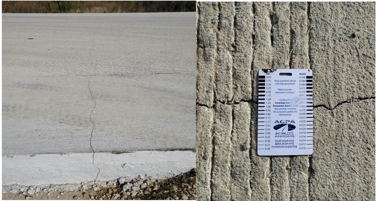
Figure 114. View of typical transverse crack in joint-free FRC overlay two weeks post-construction
